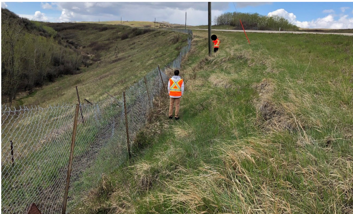
Photo 4 Slide Area 3 (east end) – The back scarp at Slide Area 3 is approximately 5 m from the south edge of the highway. The fence posts and power pole are leaning downslope towards the toe of the slope. The power pole is leaning at approximately 5° to 6° from vertical. Photo taken May 20, 2022, facing west-southwest.
