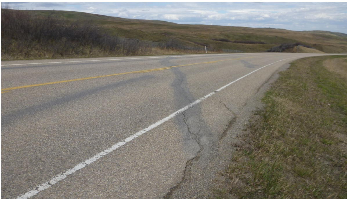
Photo 2 Sealed cracking on highway surface located approximately above the slide 2 location. Photo was taken facing north on May 10, 2019.
