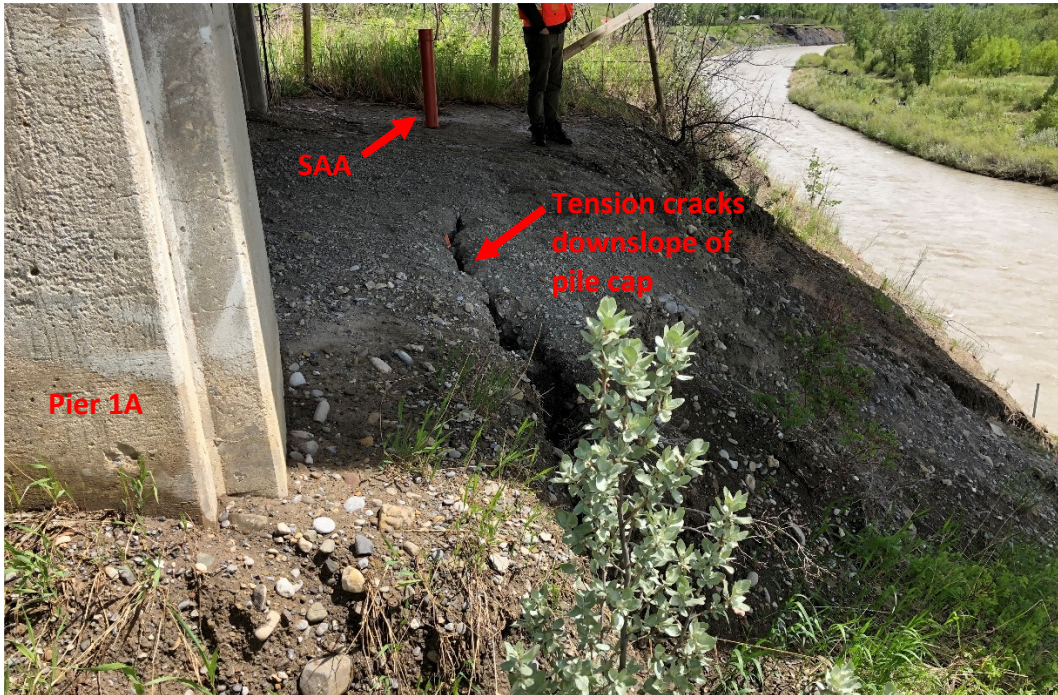
Photo 2 Tension cracking (60 to 150 mm wide) south (downslope) of the exposed Pier 1A pile cap. Photo taken facing west on June 8, 2020.
