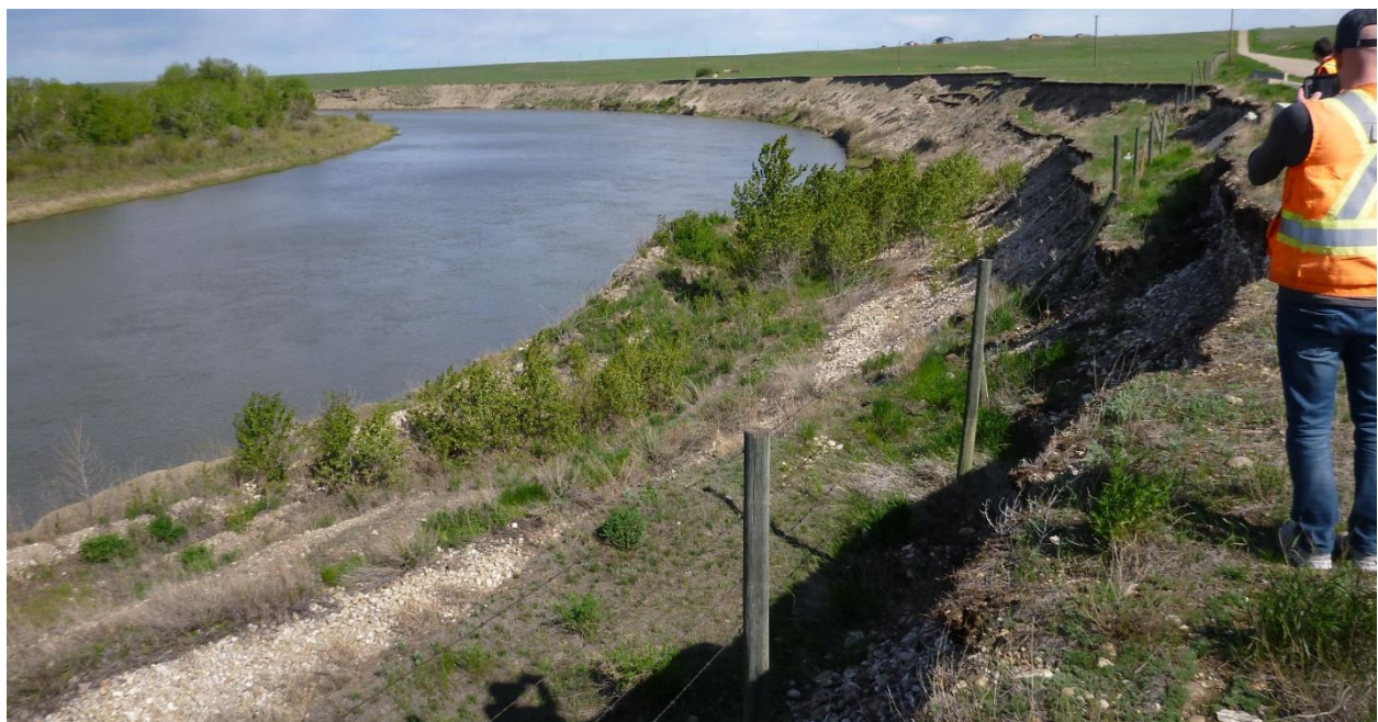
Photo 4 The head of the slide is retrogressing towards the highway and is approximately 350 m in length. The head scarp is actively eroding, and material has fallen between the 2022 and 2024 inspections. Photo taken May 29, 2024, facing north.
