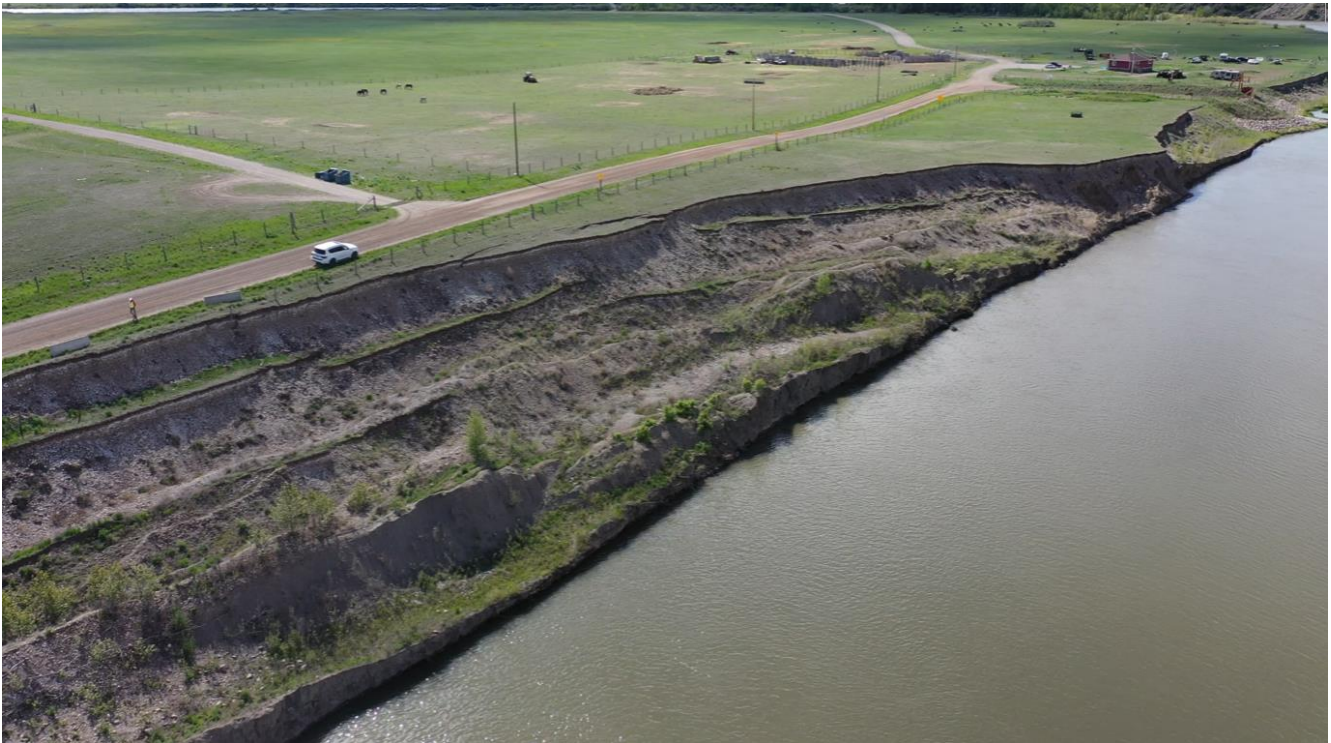
Photo 4 The head of the slide is retrogressing towards the highway and is approximately 350 m in length. The head scarp is actively eroding, and material has fallen between the 2022 and 2024 inspections. Photo taken May 29, 2024, facing north.
