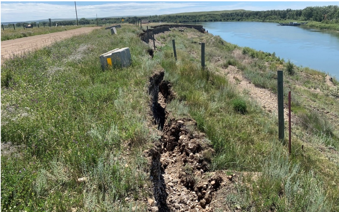
Photo 4 Six fence posts undermined by sliding. Photo taken near south end of slide facing south on July 15, 2020.
