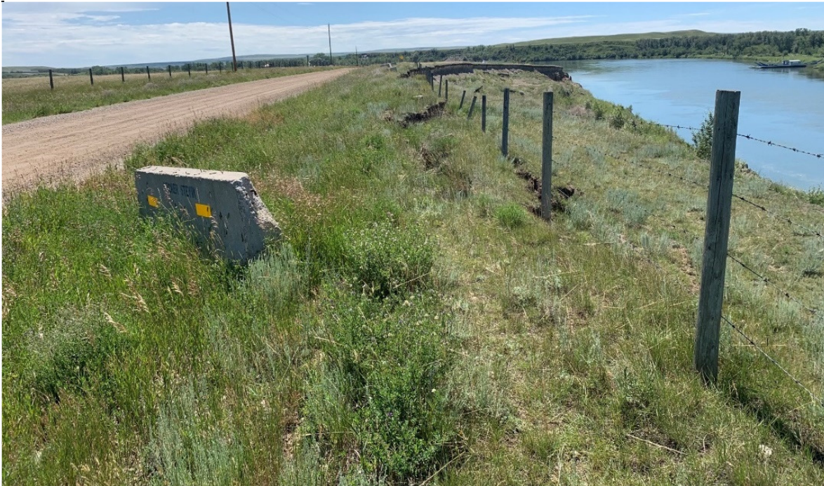
Photo 4 Six fence posts undermined by sliding. Photo taken near south end of slide facing south on July 15, 2020.
