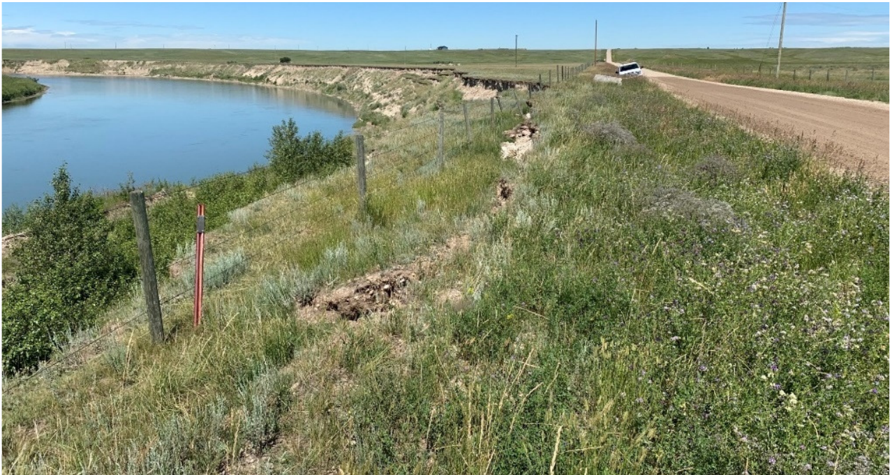
Photo 2 Tension cracking at the north end of the slide. Photo taken facing north on July 15, 2020.
