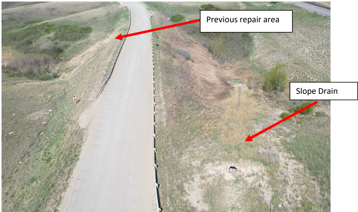
Photo 2 North side of highway – slope drain. Note exposed pipe at two locations. Photo taken facing west on May 12, 2023.
