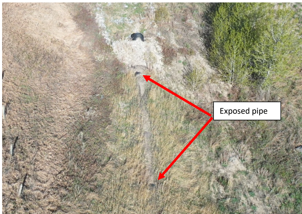
Photo 2 North side of highway – slope drain. Note exposed pipe at two locations. Photo taken facing west on May 12, 2023.
