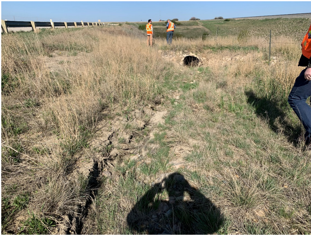
Photo 5 South side of highway – Slope failure at repair area. Red circle notes previous repair area. Photo taken facing east on May 12, 2023.
