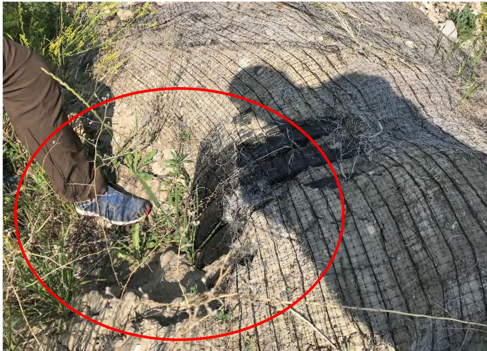
Photo 4 South side of highway – Visible granular fill and displaced vegetation near fence line due to washout of a portion of the repaired section. Photo taken on July 7, 2021.
