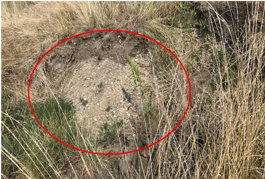
Photo 4 South side of highway – Visible granular fill and displaced vegetation near fence line due to washout of a portion of the repaired section. Photo taken on July 7, 2021.
