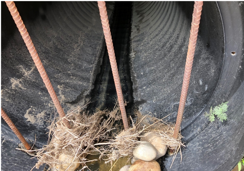
Photo 2 Flow in the HDPE pipe. The volume of flow in the slope drain appeared to be lower than the volume of flow in the ditch. Photo taken on July 8, 2020.
