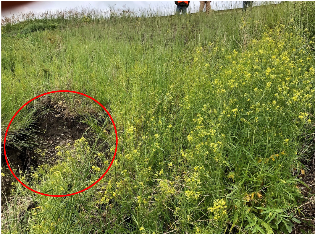
Photo 6 South side of highway – Recent failure at the toe of the repaired section (previously repaired in 2018). Photo taken facing south on July 8, 2020.
