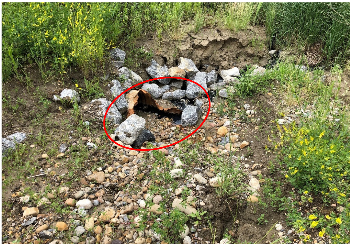
Photo 4 North side of highway – Culvert under highway remains blocked with sediment due to 2019 ditch block overtopping. Photo taken facing south on July 8, 2020.
