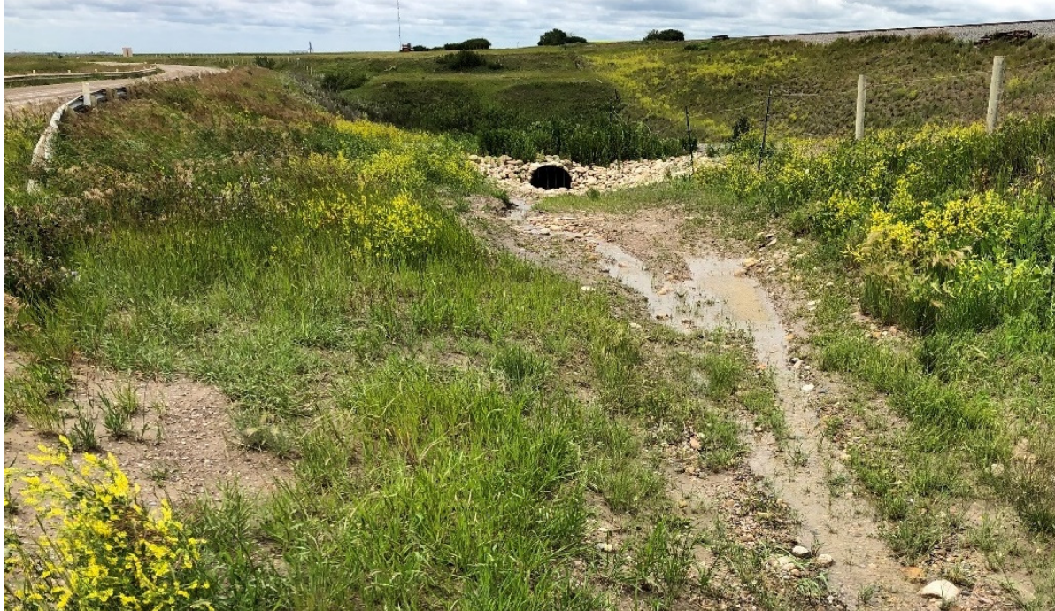
Photo 2 Flow in the HDPE pipe. The volume of flow in the slope drain appeared to be lower than the volume of flow in the ditch. Photo taken on July 8, 2020.
