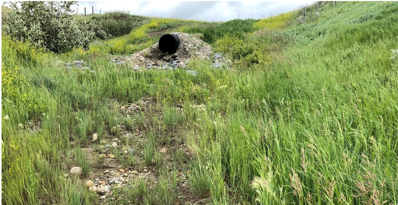
Photo 4 North side of highway – Culvert under highway remains blocked with sediment due to 2019 ditch block overtopping. Photo taken facing south on July 8, 2020.
