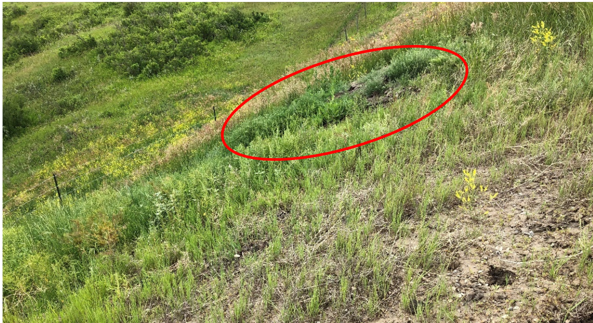
Photo 6 South side of highway – Recent failure at the toe of the repaired section (previously repaired in 2018). Photo taken facing south on July 8, 2020.
