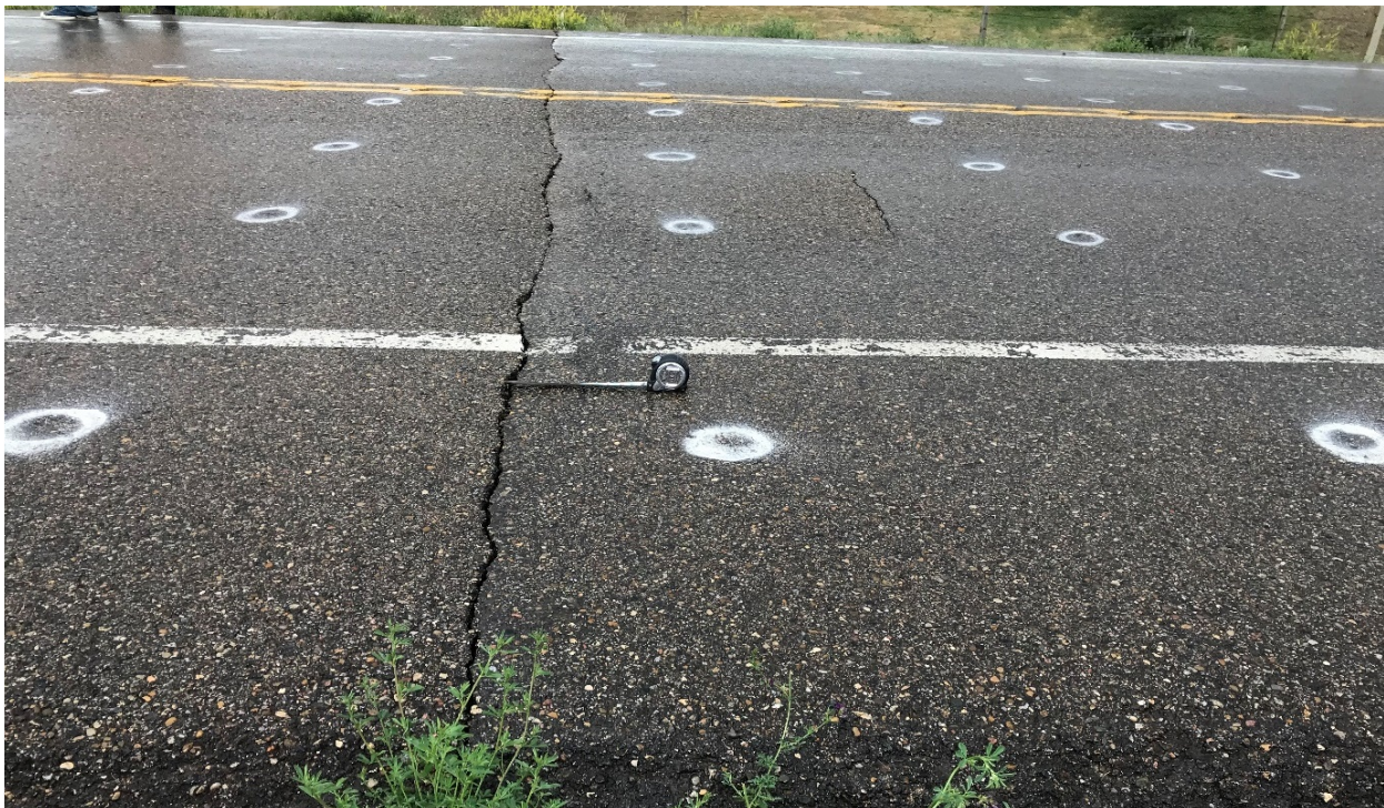
Photo 2 Full pavement depth transverse crack at the dip. Crack is up to 2 cm wide. White circles denote survey pins installed in a grid pattern. Photo was taken facing north on July 8, 2021.
