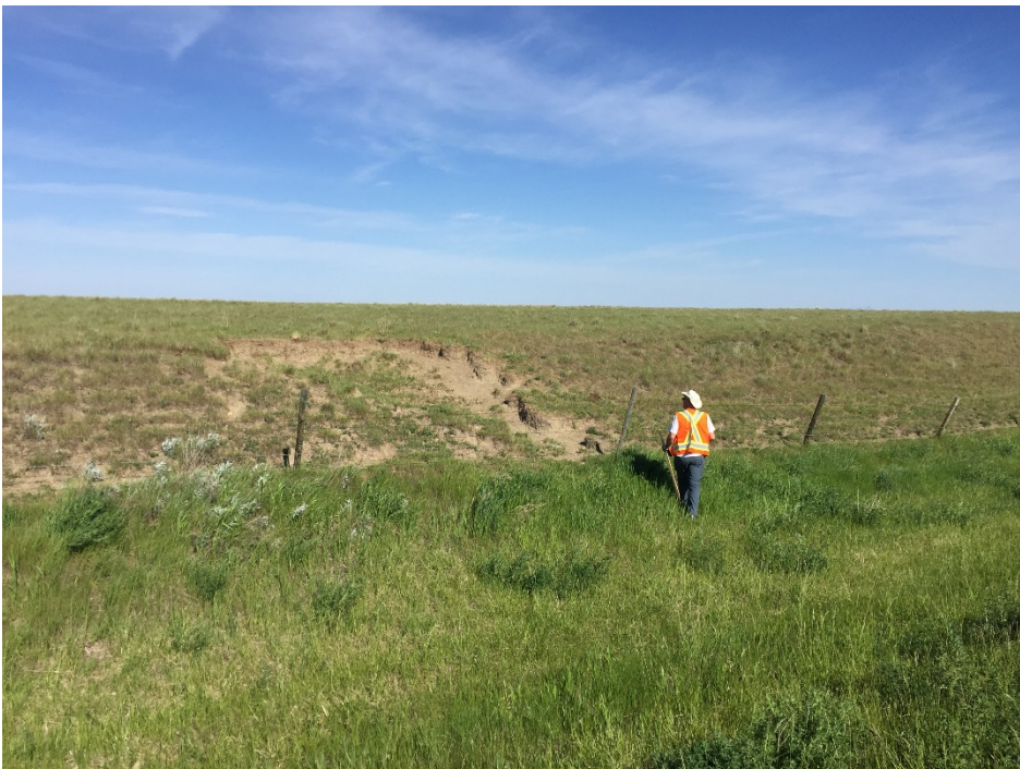
Photo 4 Depression/erosion feature on the west side of the highway. Photo was taken facing west on May 31, 2017.
