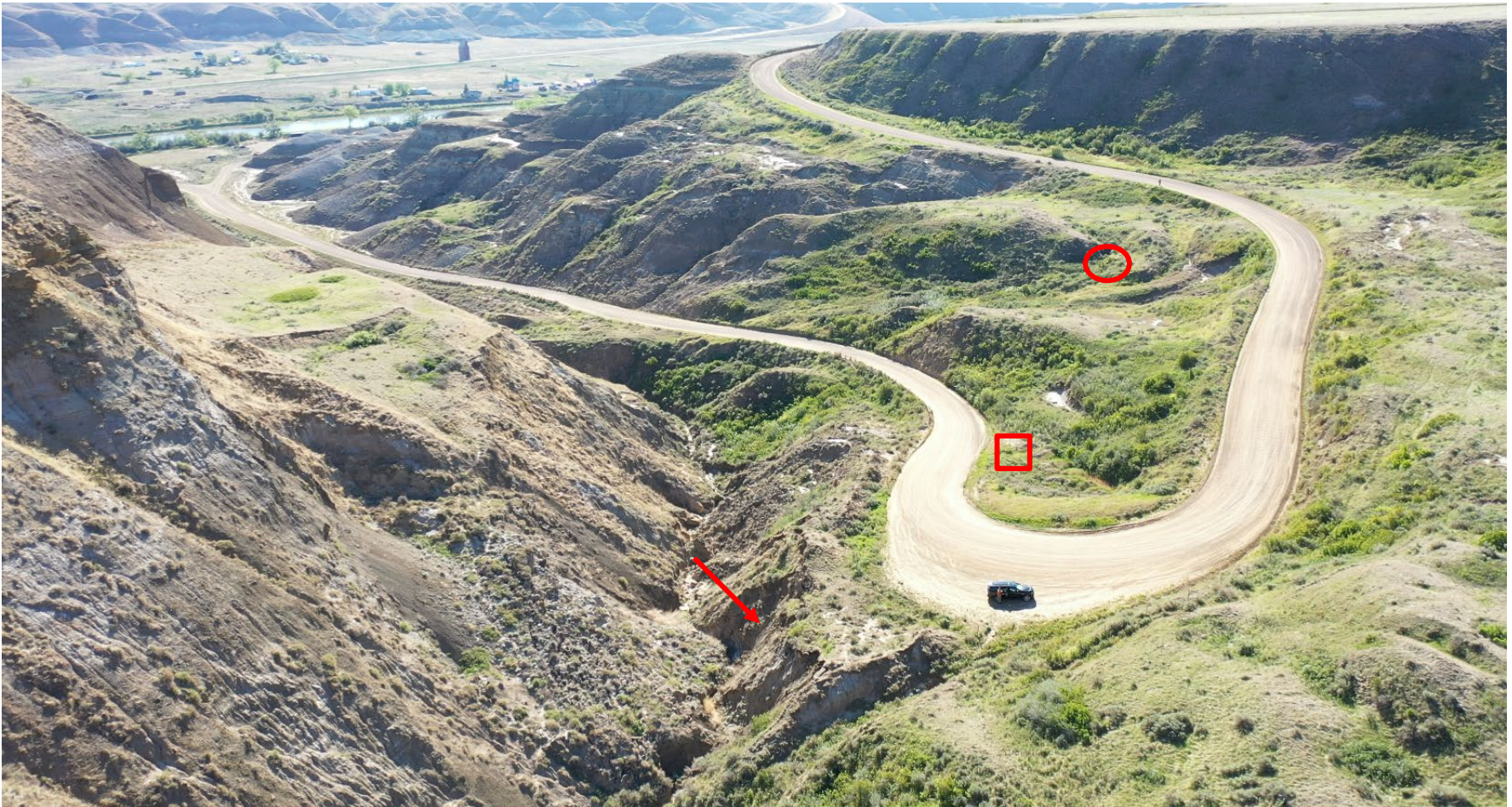
Photo 1 An aerial photo of the S040 Dorothy Sinkholes site. The erosion on the ditch slope, approximate location of the culvert inlet, and a large new sinkhole (WP 164) are indicated by a red arrow, square, and circle, respectively. The highway was graded shortly before the 2022 inspection. Photo taken May 31, 2022, facing east.
