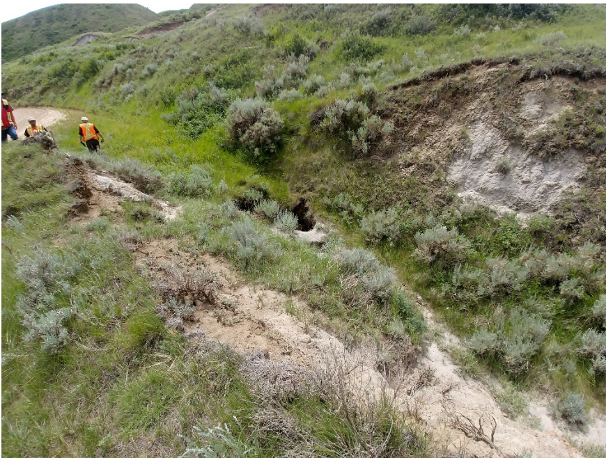
Photo 2 Existing erosion gully and void directly west of hairpin curve. Photo taken July 10, 2019 looking south.
