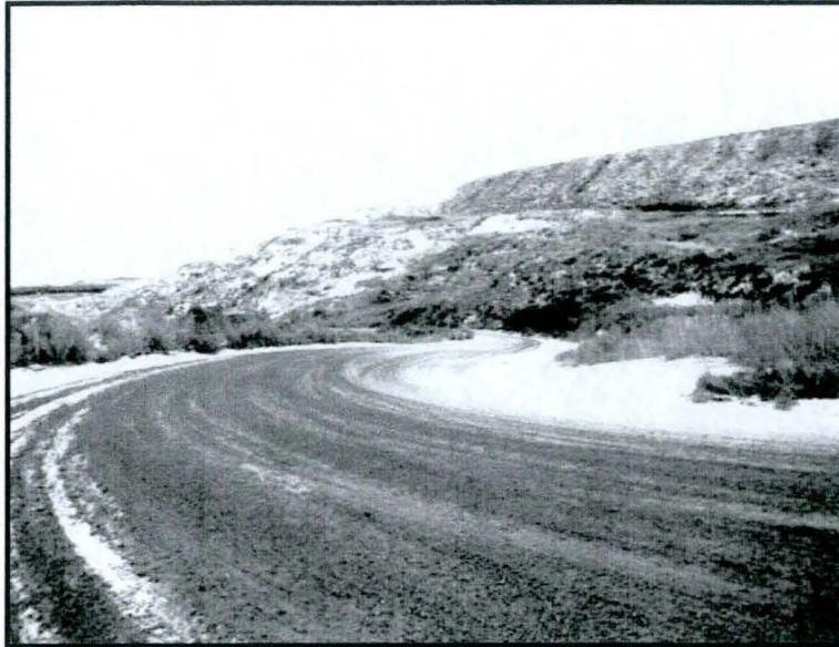
Photo 1 (left) Standing at the hairpin turn where previous sinkhole damage was reported by the MCI. Facing towards the east. (Photo Date: November 21, 2011)
