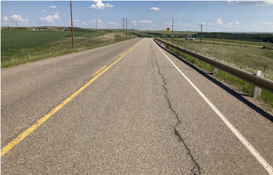
Photo 4 The west highway embankment slope and S046-I and -III repairs are well vegetated and appear to be performing well. The fence near the embankment toe is deflected towards the west, and may be attributed to slope movement before construction, or settlement of the repair fill. Photo taken June 26, 2023, facing north.
