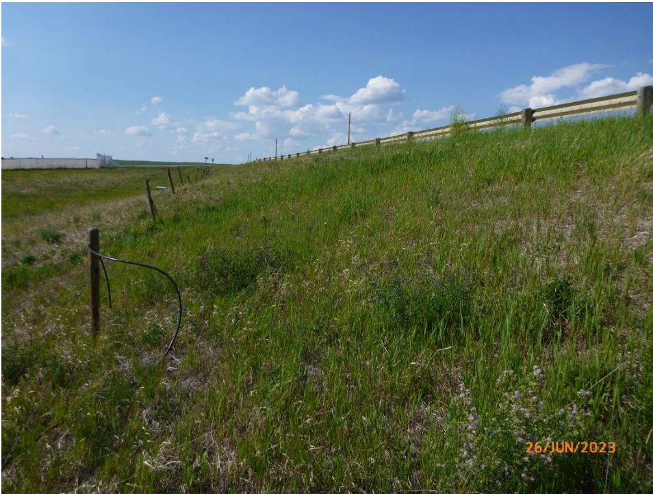
Photo 4 The west highway embankment slope and S046-I and -III repairs are well vegetated and appear to be performing well. The fence near the embankment toe is deflected towards the west, and may be attributed to slope movement before construction, or settlement of the repair fill. Photo taken June 26, 2023, facing north.
