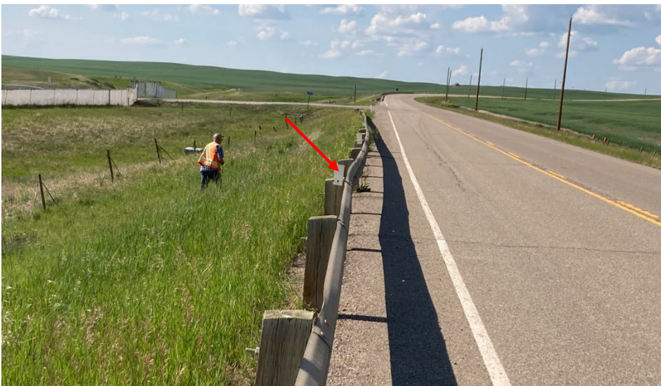
Photo 2 Minor guardrail deflection (indicated by red arrow) upslope of S046-I, most likely attributed to a vehicle accident or road maintenance activities since the 2019 inspection. Photo taken June 26, 2023, facing north.
