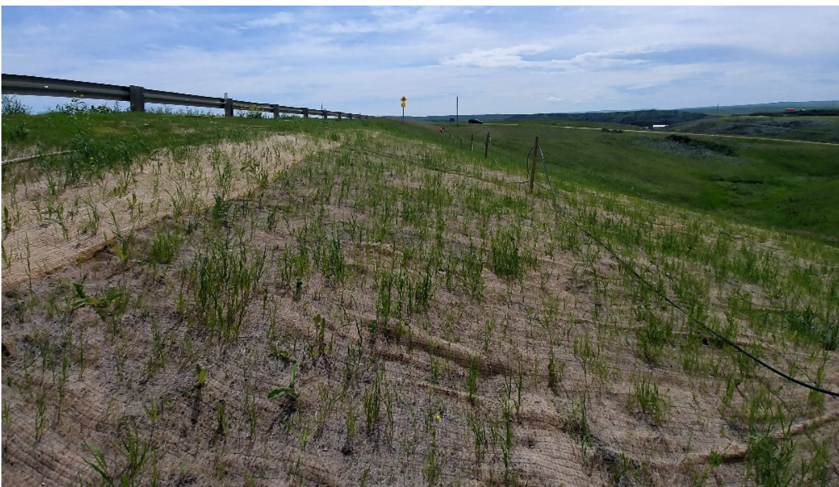
Photo 2 Close-up view of S046-III slide repair and erosion control blanket. Photo taken July 10, 2019 looking southeast.
