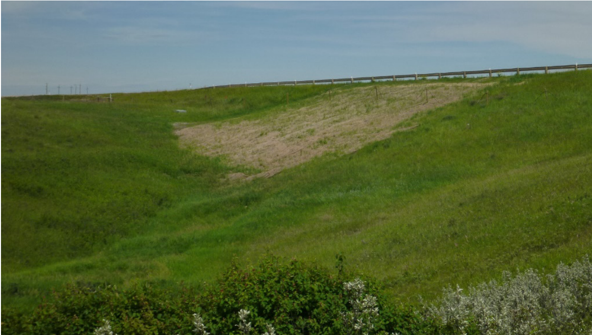
Photo 2 Close-up view of S046-III slide repair and erosion control blanket. Photo taken July 10, 2019 looking southeast.
