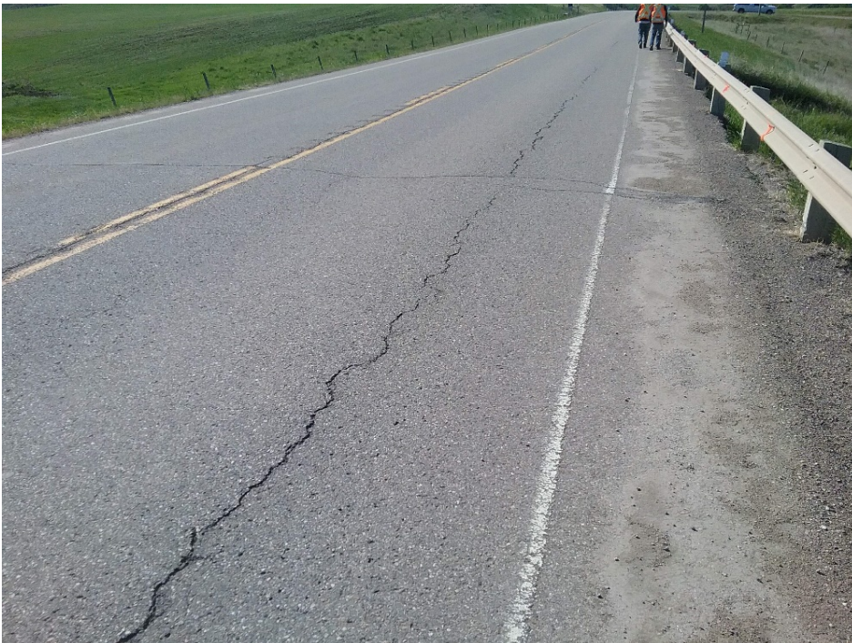
Photo 2 Condition of pavement at head of slide. Photo taken June 12, 2018 looking south.
