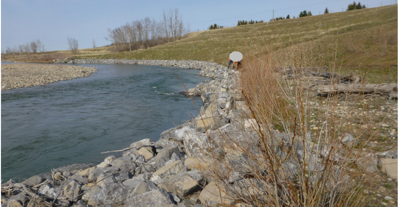
Photo 4 Erosion at upstream limit of riprap. Minimal change noted from previous inspection. Photo was taken facing east on May 9, 2019.
