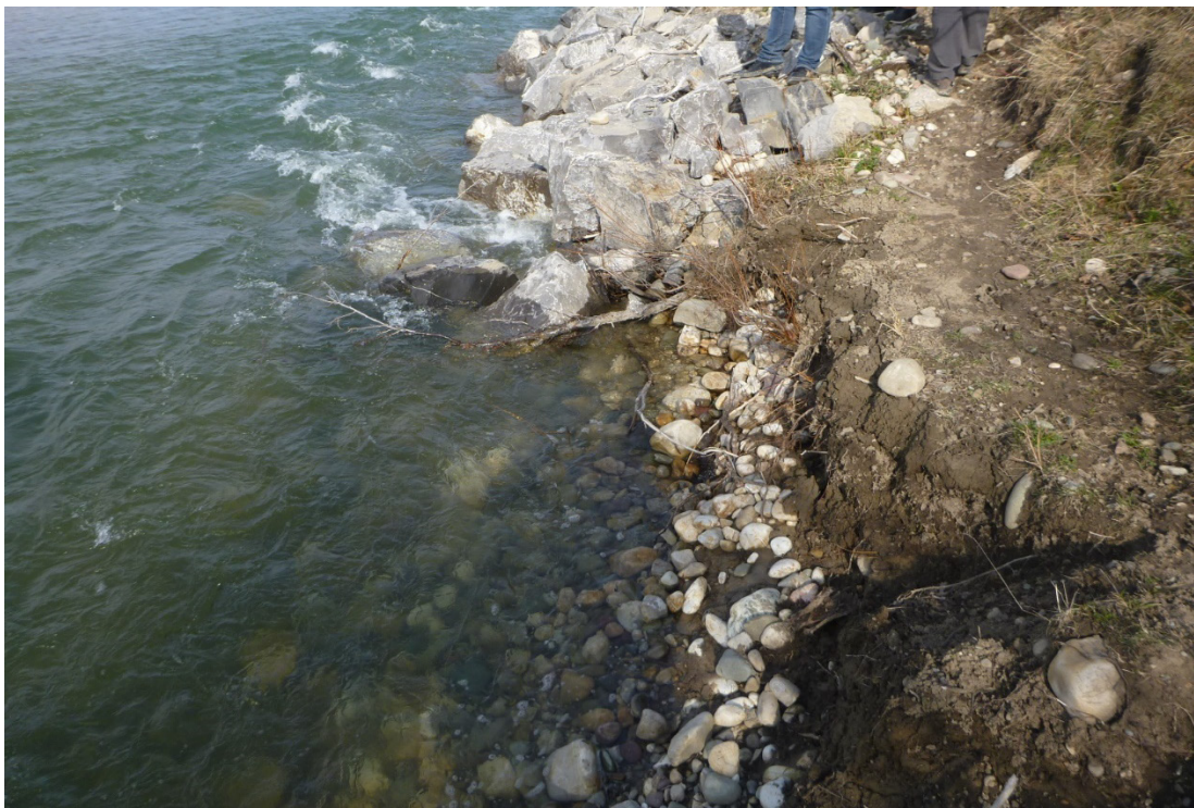
Photo 4 Erosion at upstream limit of riprap. Minimal change noted from previous inspection. Photo was taken facing east on May 9, 2019.
