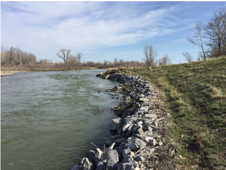
Photo 4 North toe area of repaired slide area. Some rip rap has been displaced from the re-directive vanes at river edge. Photo was taken facing north on May 3, 2018.
