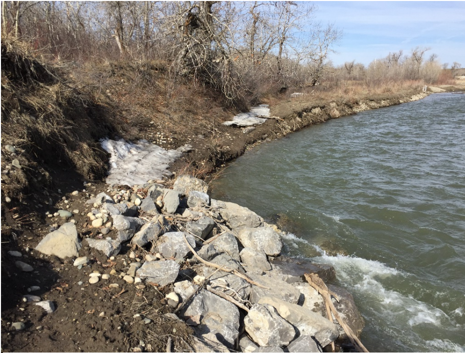
Photo 4 North toe area of repaired slide area. Some rip rap has been displaced from the re-directive vanes at river edge. Photo was taken facing north on May 3, 2018.
