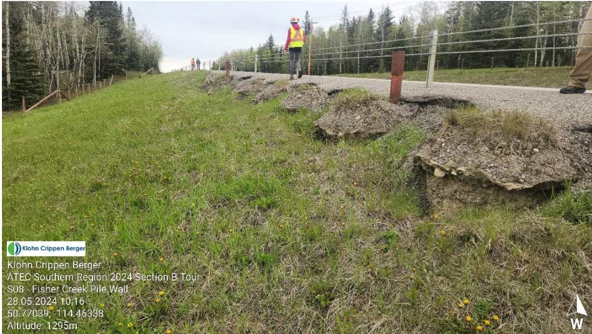
Photo 4 Settlement downslope of pile wall, exposed concrete pilea. Photo taken facing southeast on May 28, 2024.
