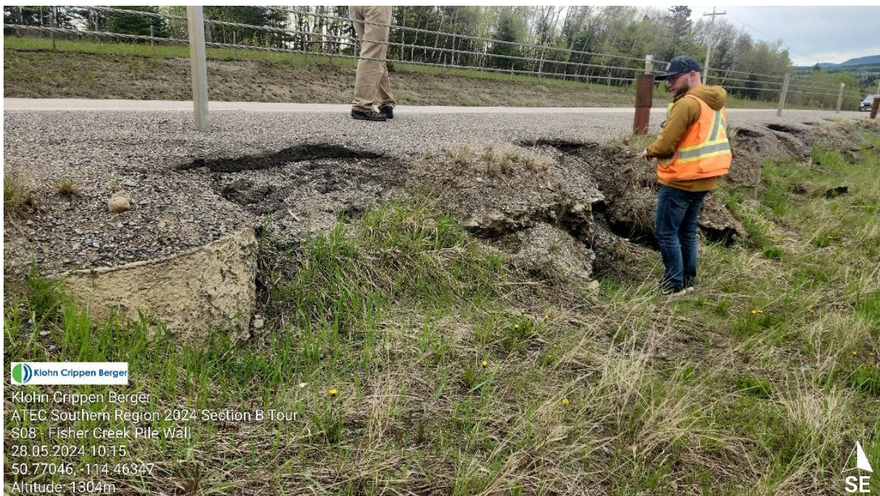
Photo 4 Settlement downslope of pile wall, exposed concrete pilea. Photo taken facing southeast on May 28, 2024.
