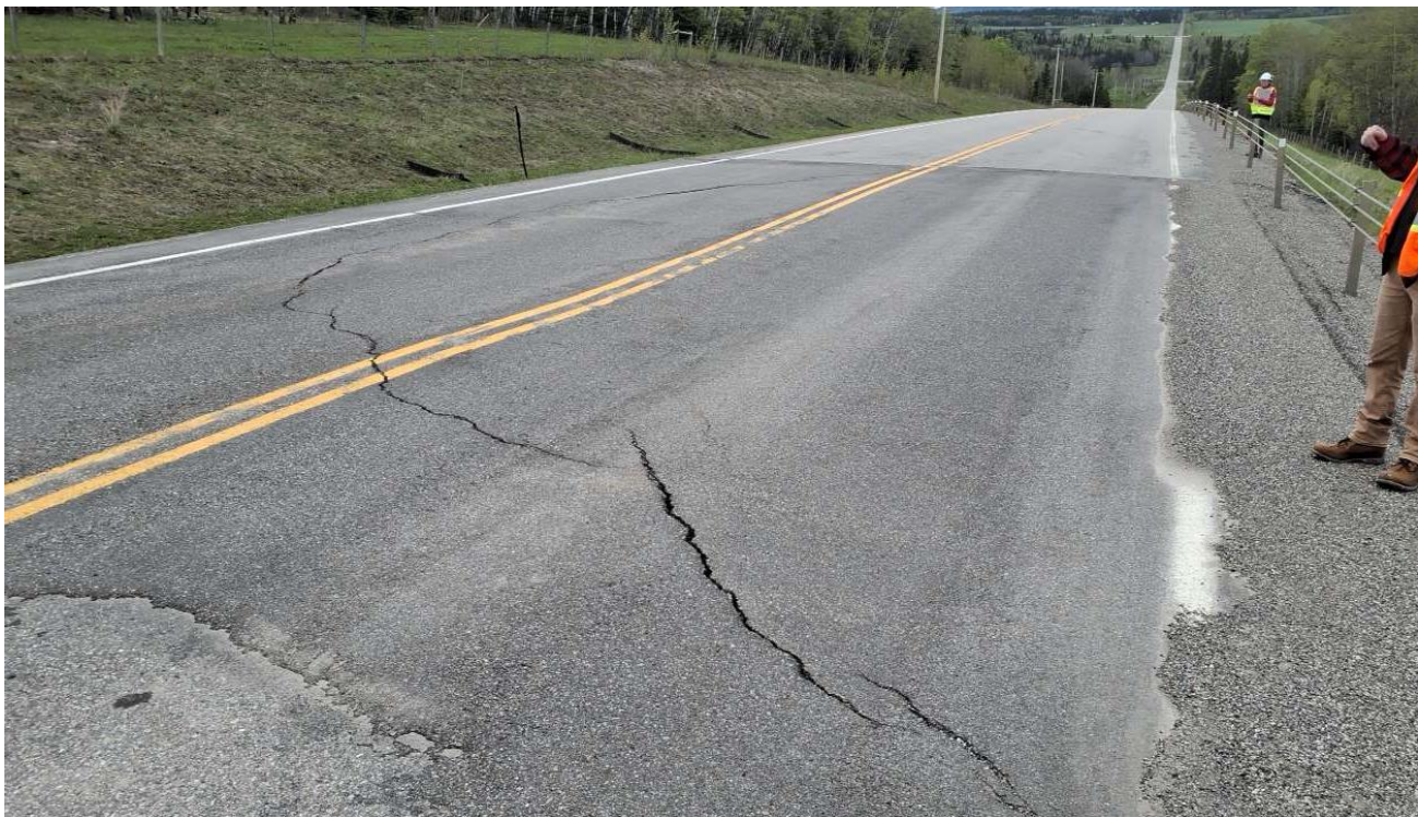
Photo 2 Cracking in the northbound lane. Photo taken facing south on May 28, 2024
