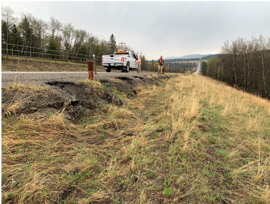
Photo 4 Settlement downslope of pile wall. Photo taken facing south on May 9, 2023.
