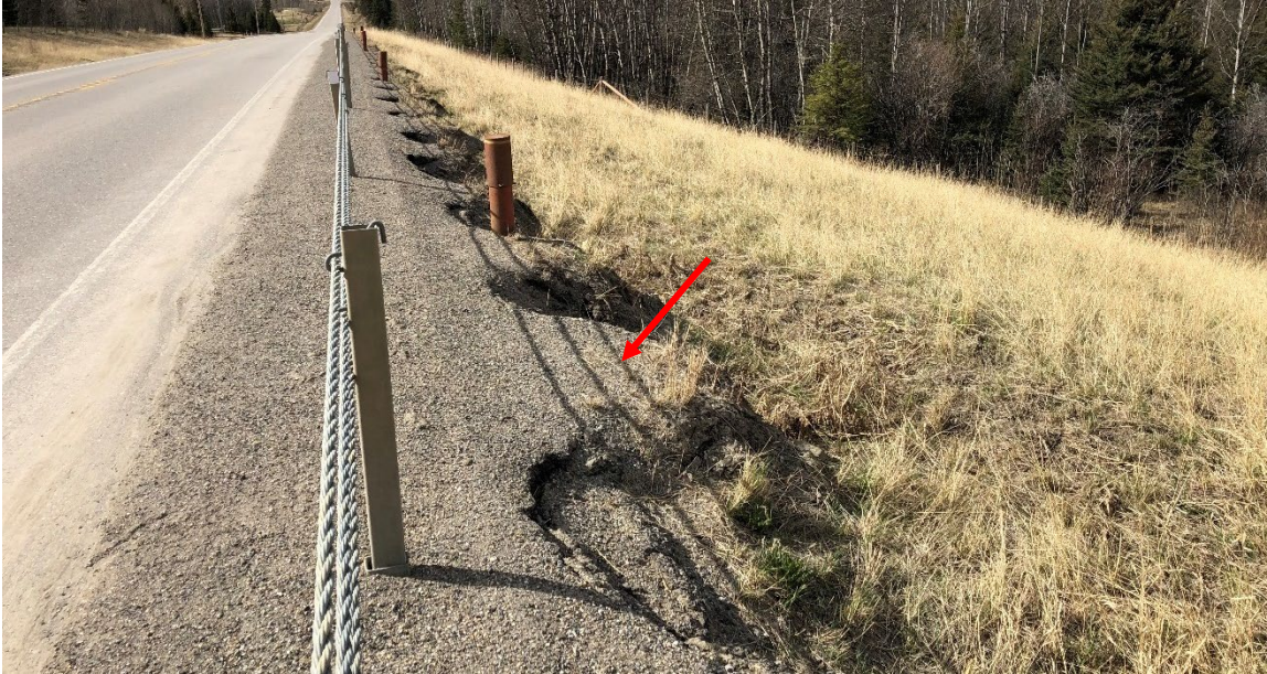
Photo 4 There has been approximately 600 mm of settlement of embankment fill downslope of the pile wall. Photo taken on May 16, 2022, facing north east.
