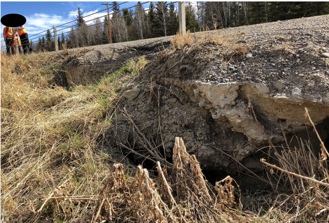
Photo 4 There has been approximately 600 mm of settlement of embankment fill downslope of the pile wall. Photo taken on May 16, 2022, facing north east.
