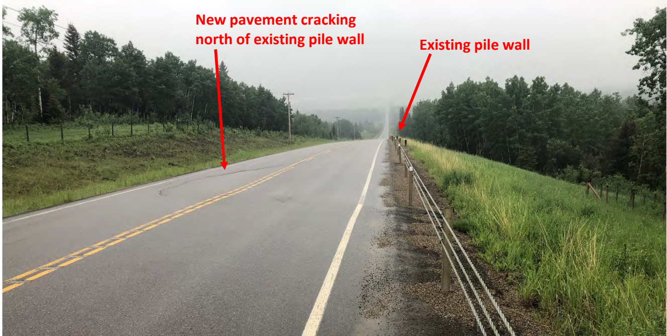
Photo 2 Pavement cracking in the northbound lane, north of the existing pile wall. Photo taken facing south on July 5, 2021.
