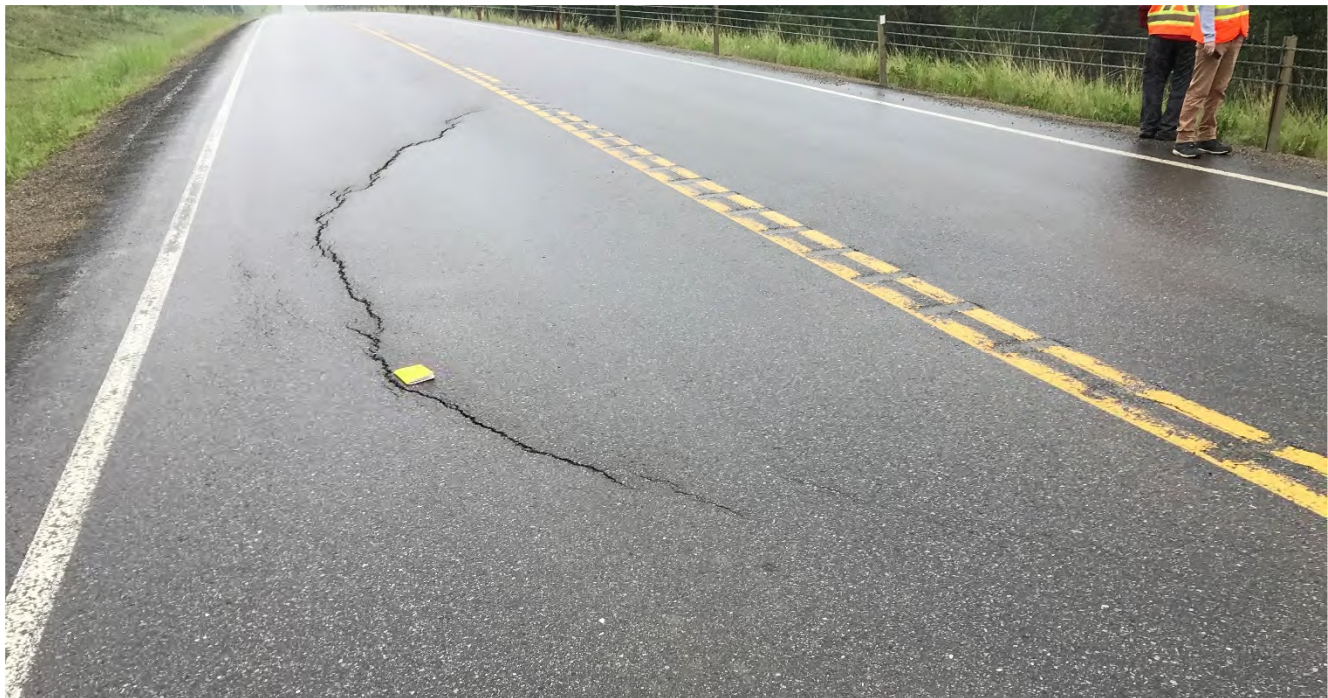
Photo 2 Pavement cracking in the northbound lane, north of the existing pile wall. Photo taken facing south on July 5, 2021.
