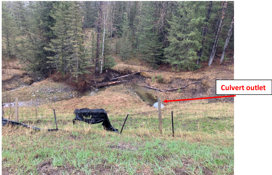
Photo 2 Toe erosion and fence deflection on embankment slope. Photo taken facing northeast on May 9, 2023.
