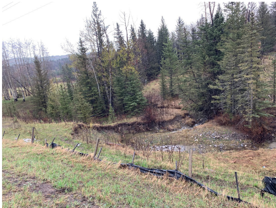
Photo 2 Toe erosion and fence deflection on embankment slope. Photo taken facing northeast on May 9, 2023.
