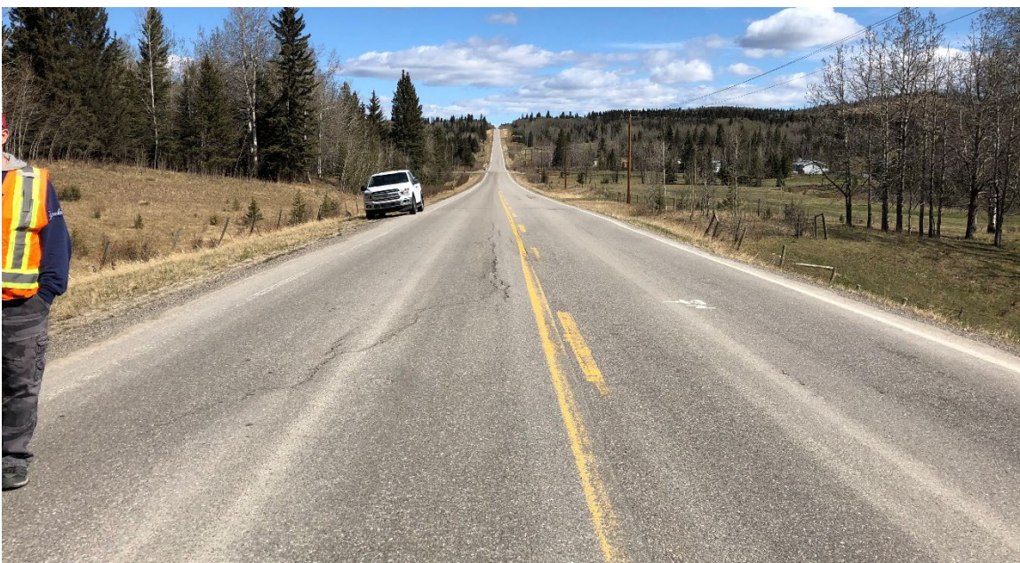
Photo 4 Longitudinal pavement cracking in the west (southbound) lane. Photo taken May 16, 2022, facing north.
