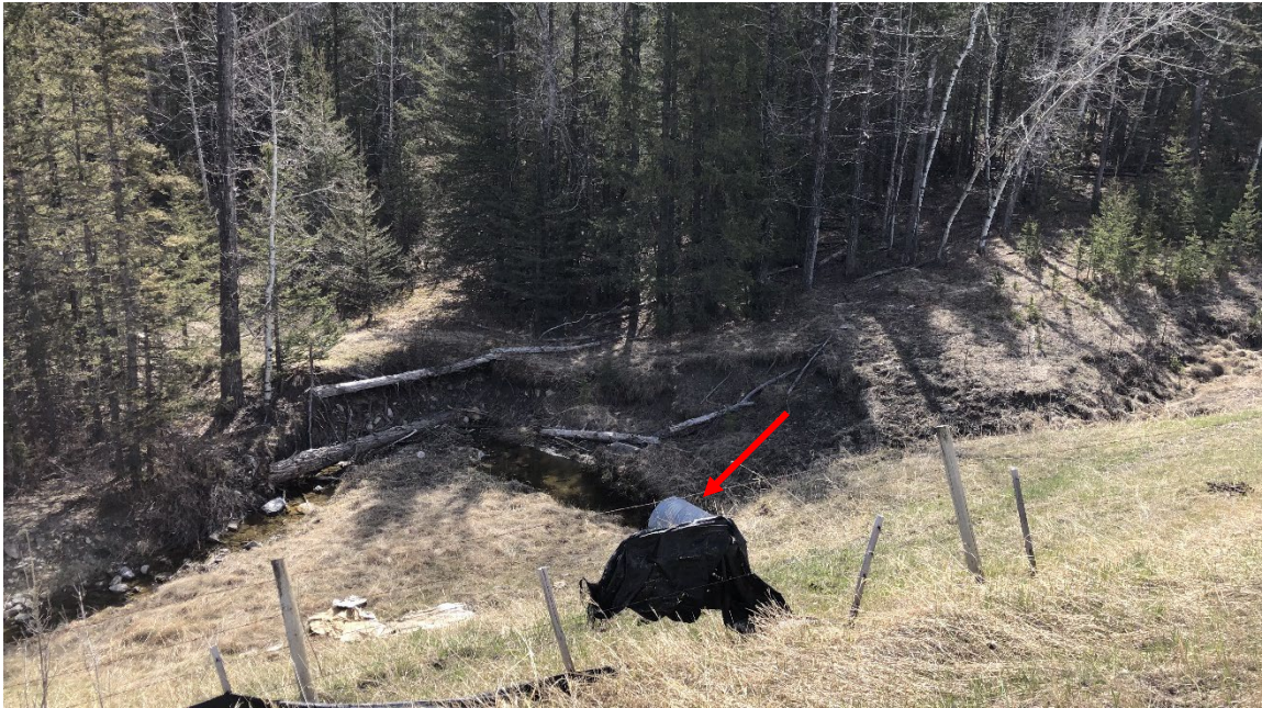
Photo 2 Toe erosion and fence deflection on east highway embankment slope. CSP culvert outlet is indicated by red arrow. Photo taken May 16, 2022, facing north.
