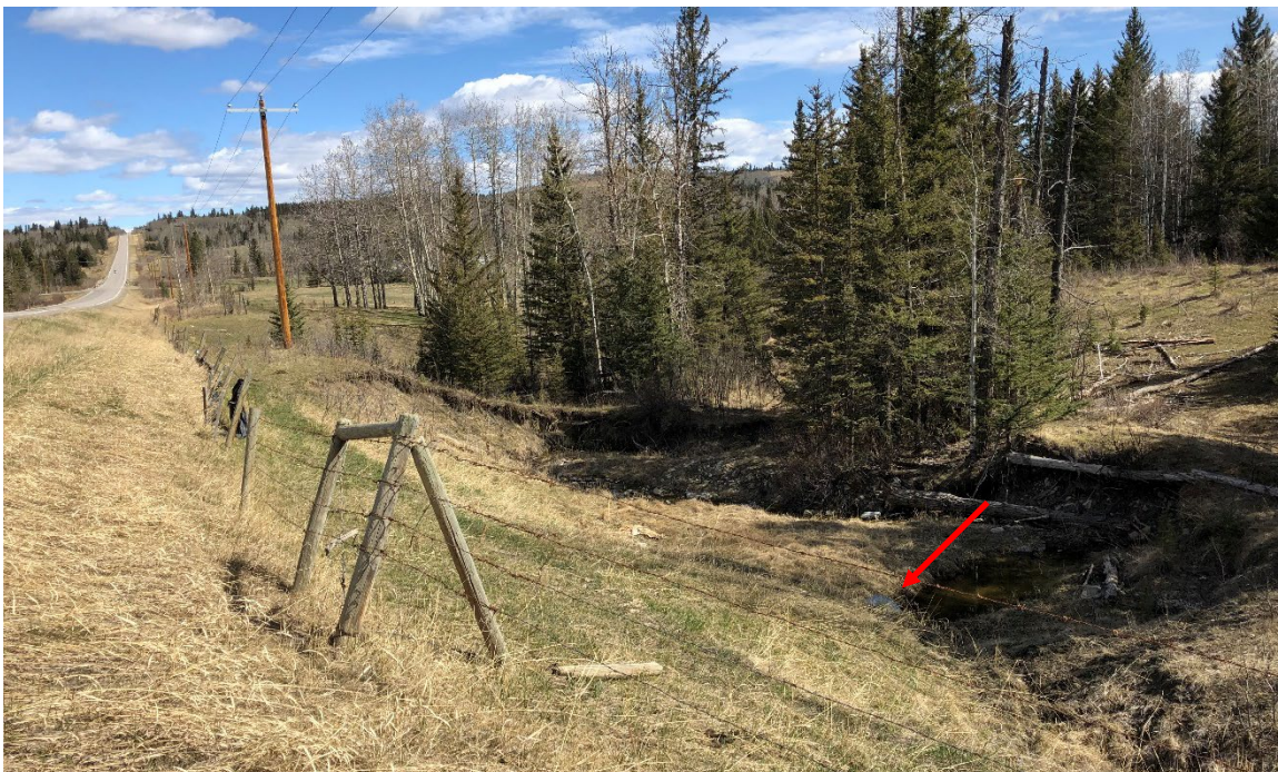
Photo 2 Toe erosion and fence deflection on east highway embankment slope. CSP culvert outlet is indicated by red arrow. Photo taken May 16, 2022, facing north.
