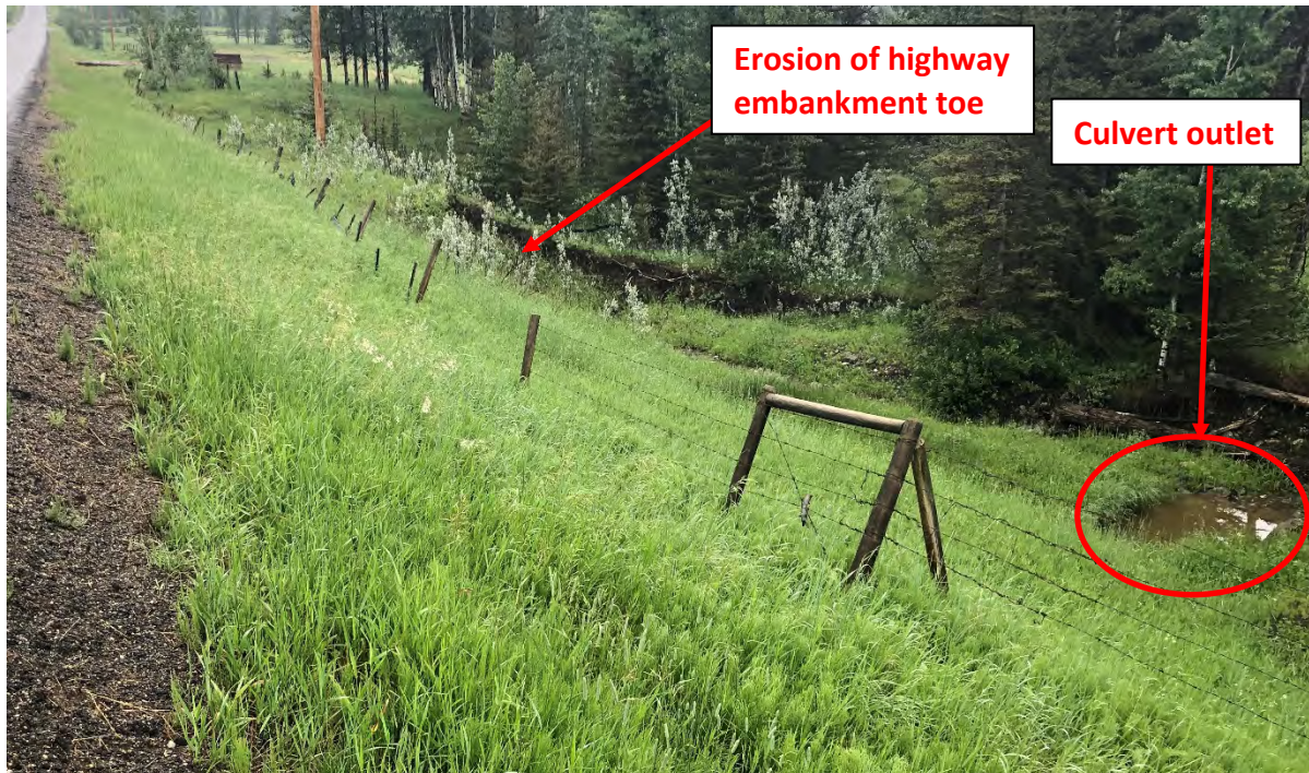
Photo 2 Toe erosion and fence deflection on embankment slope. Photo taken facing north on July 5, 2021.
