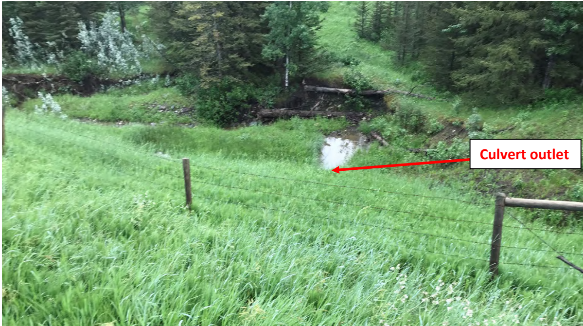
Photo 2 Toe erosion and fence deflection on embankment slope. Photo taken facing north on July 5, 2021.
