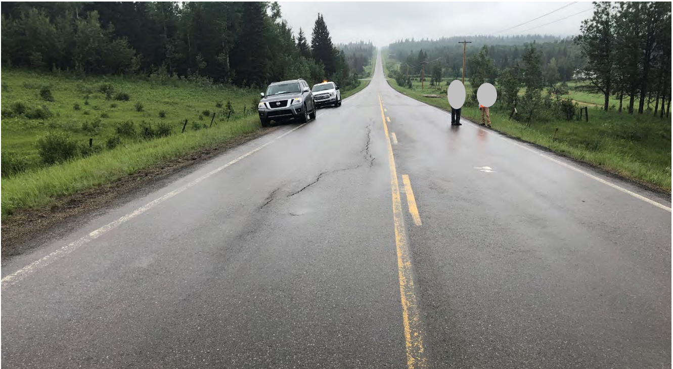
Photo 4 Longitudinal pavement cracking. Photo was taken facing south on July 5, 2021.
