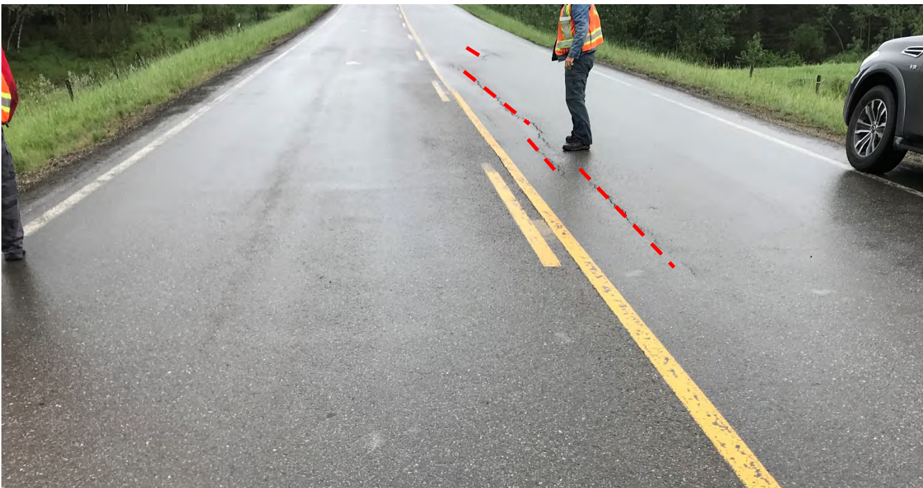
Photo 4 Longitudinal pavement cracking. Photo was taken facing south on July 5, 2021.
