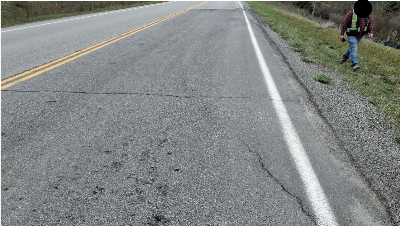
Photo 4 Cracking on the shoulder of the southbound lane. Photo on May 28, 2024
