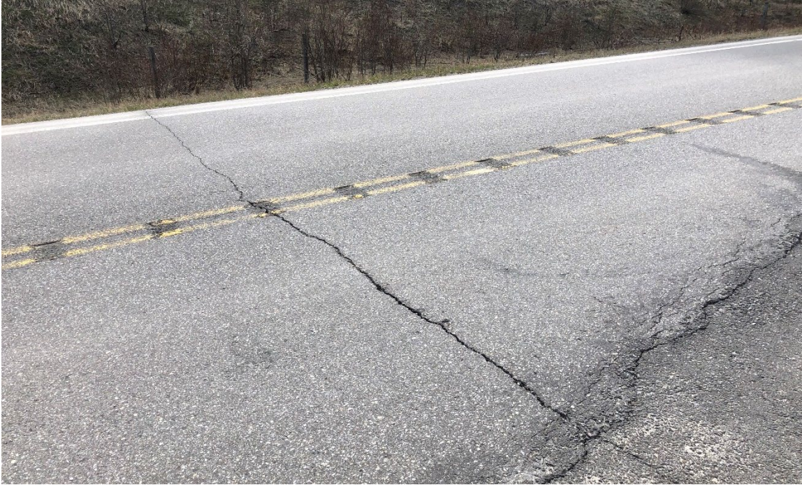
Photo 4 Longitudinal pavement crack in the west (southbound) lane. Photo taken May 16, 2022, facing east.
