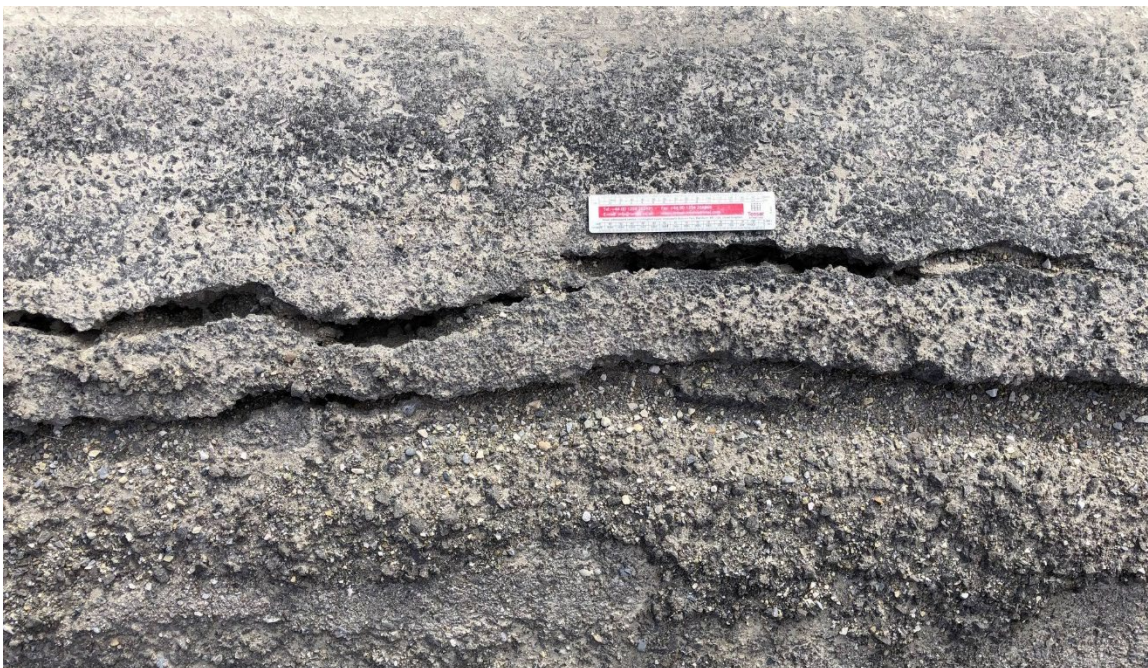
Photo 4 Longitudinal pavement crack in the west (southbound) lane. Photo taken May 16, 2022, facing east.
