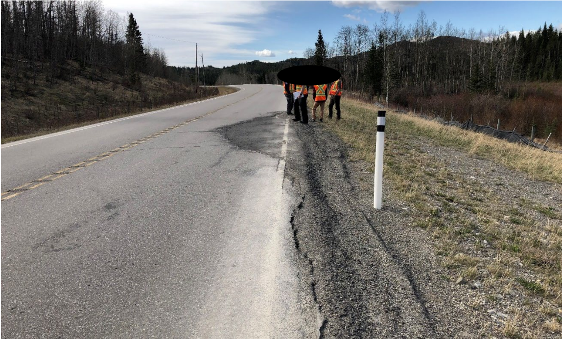
Photo 2 Pavement patch north of the slide repair area where there has been pavement cracking and settlement. Photo was taken May 16, 2022, facing southeast.
