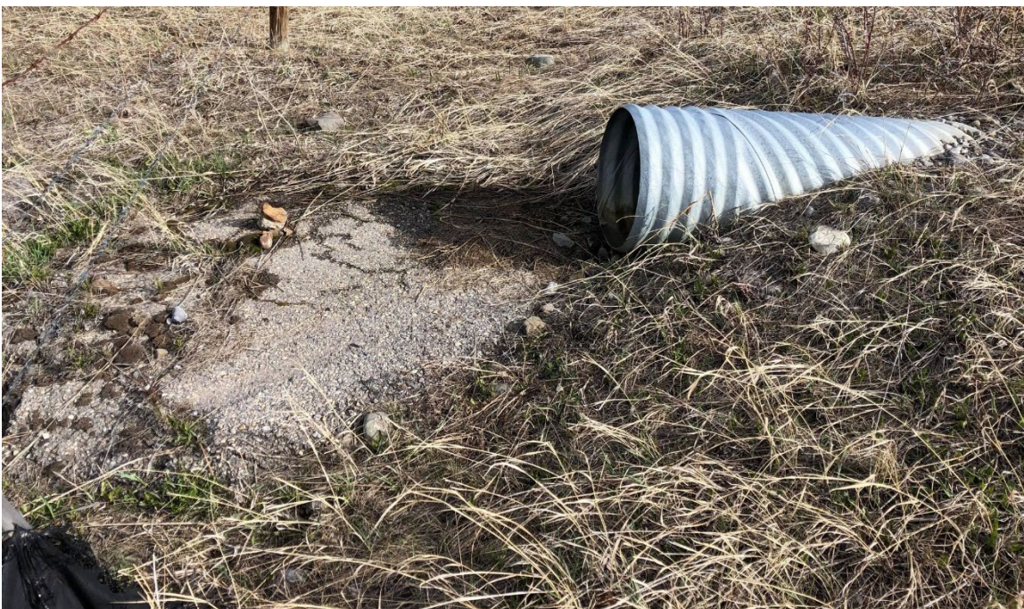
Photo 6 Asphalt apron at the outlet of the north CSP culvert. Photo taken May 16, 2022, facing north.
