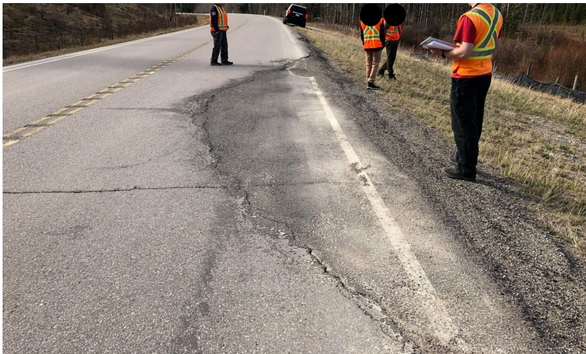
Photo 2 Pavement patch north of the slide repair area where there has been pavement cracking and settlement. Photo was taken May 16, 2022, facing southeast.
