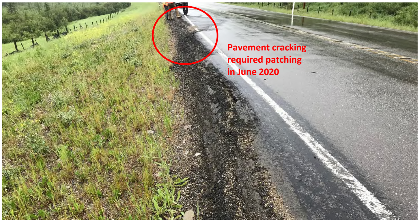
Photo 2 S031 Site II – Pavement cracking north of slide repair. Photo was taken facing southwest on July 5, 2021.
