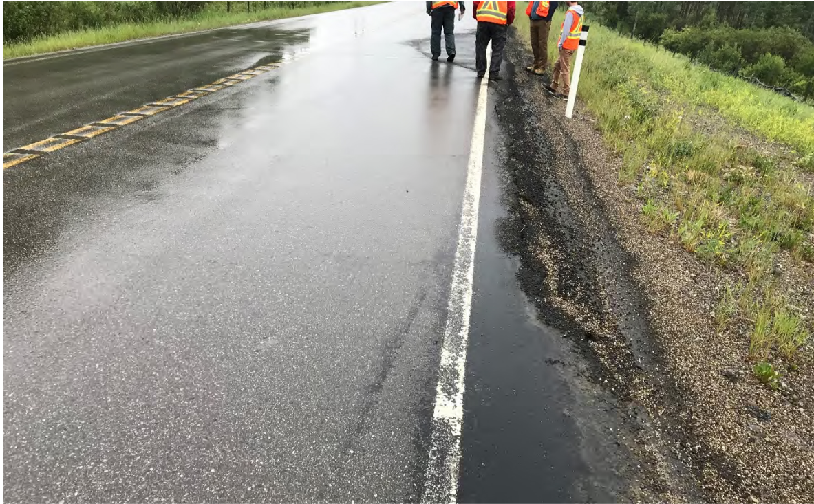
Photo 2 S031 Site II – Pavement cracking north of slide repair. Photo was taken facing southwest on July 5, 2021.
