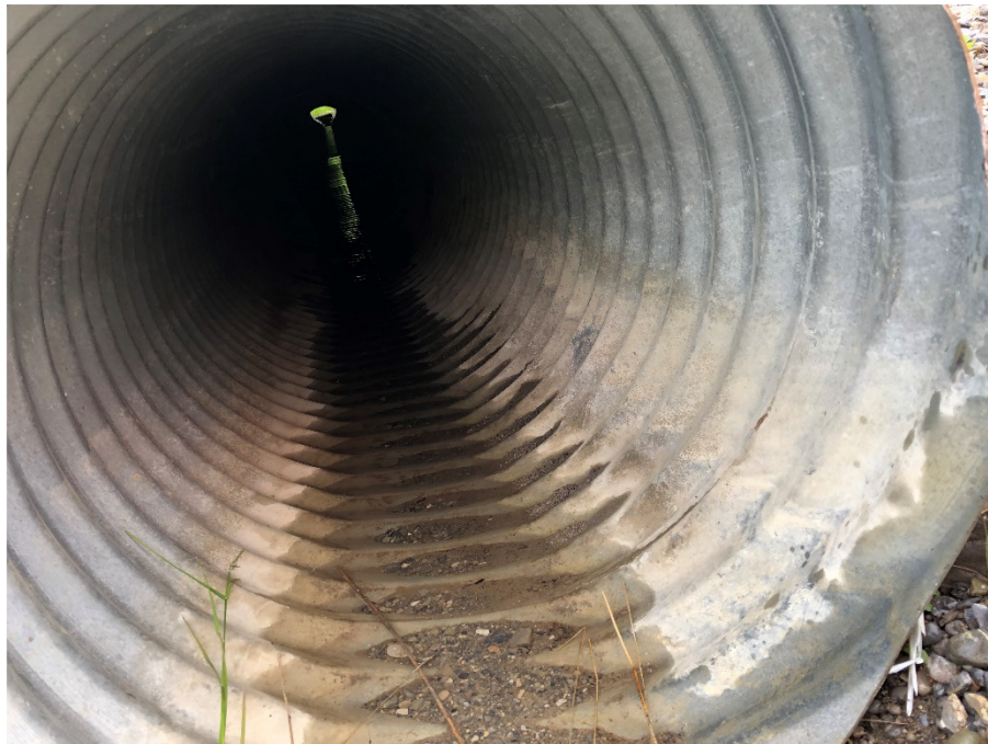
Photo 4 S031 Site II – Culvert appears bowed beneath highway. Photo was taken facing east on July 8, 2020.
