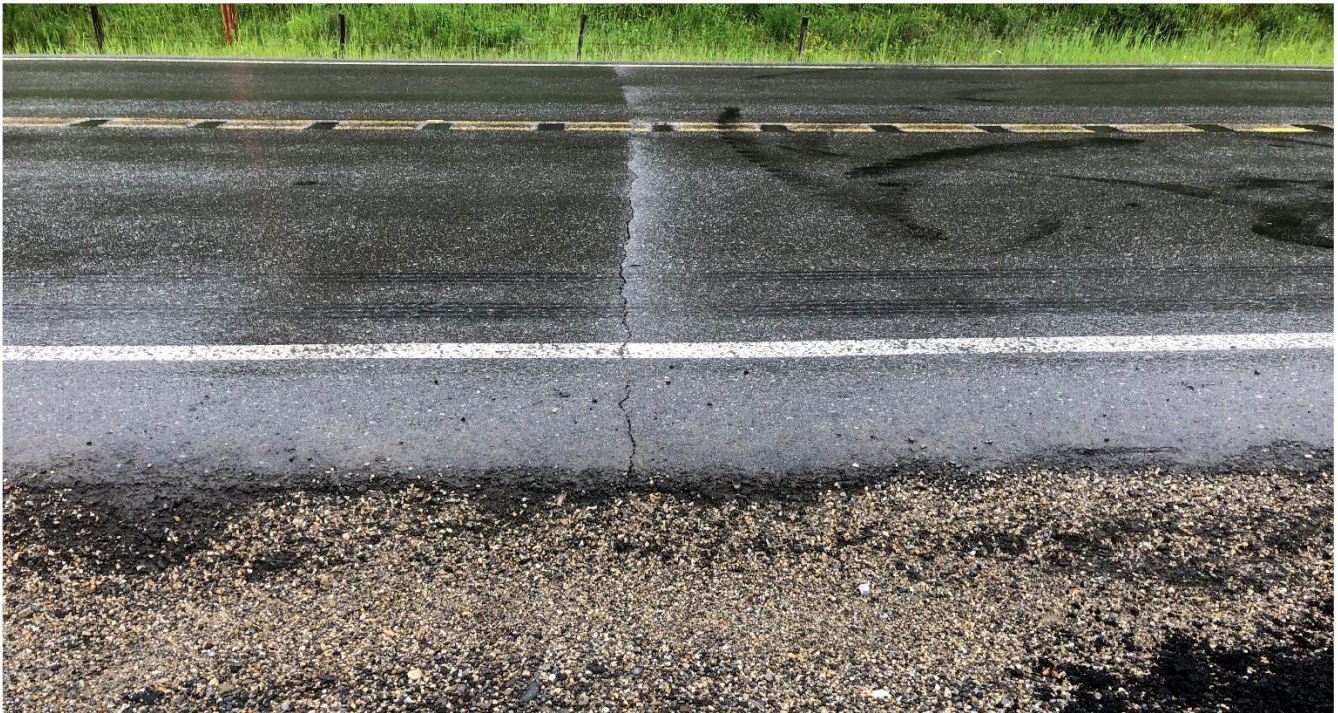
Photo 4 S031 Site II – Culvert appears bowed beneath highway. Photo was taken facing east on July 8, 2020.
