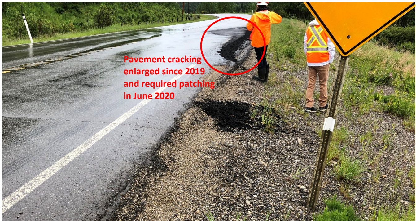
Photo 2 S031 Site II – Pavement cracking north of slide repair. Photo was taken facing east on July 8, 2020.
