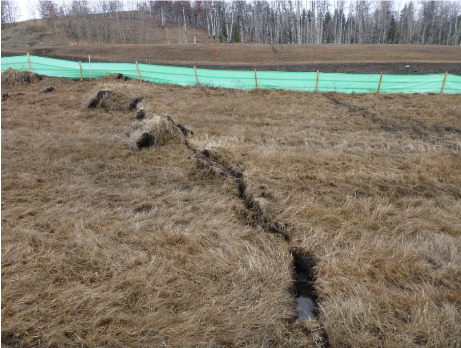
Photo 4 Cracking in field south of highway. Cracks noted to extend about 50 m into the field from highway. Photo taken facing south on April 30, 2018.
