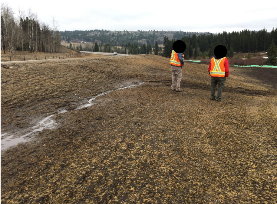
Photo 2 Surface water from ditch draining into adjacent field, causing erosion. Vegetation not established at time of inspection. Photo taken facing southeast on April 30, 2018.
