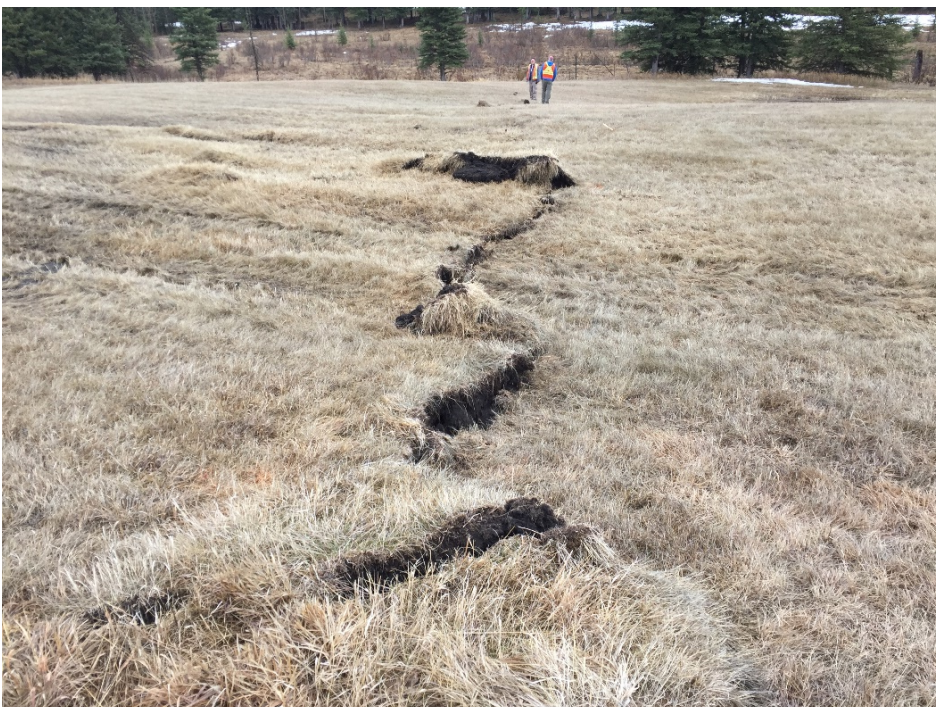
Photo 4 Cracking in field south of highway. Cracks noted to extend about 50 m into the field from highway. Photo taken facing south on April 30, 2018.
