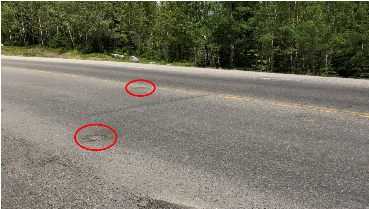
Photo 2 Pavement cracking and flush-mounted headbox for old boreholes. Photo taken facing west on July 6, 2020.
