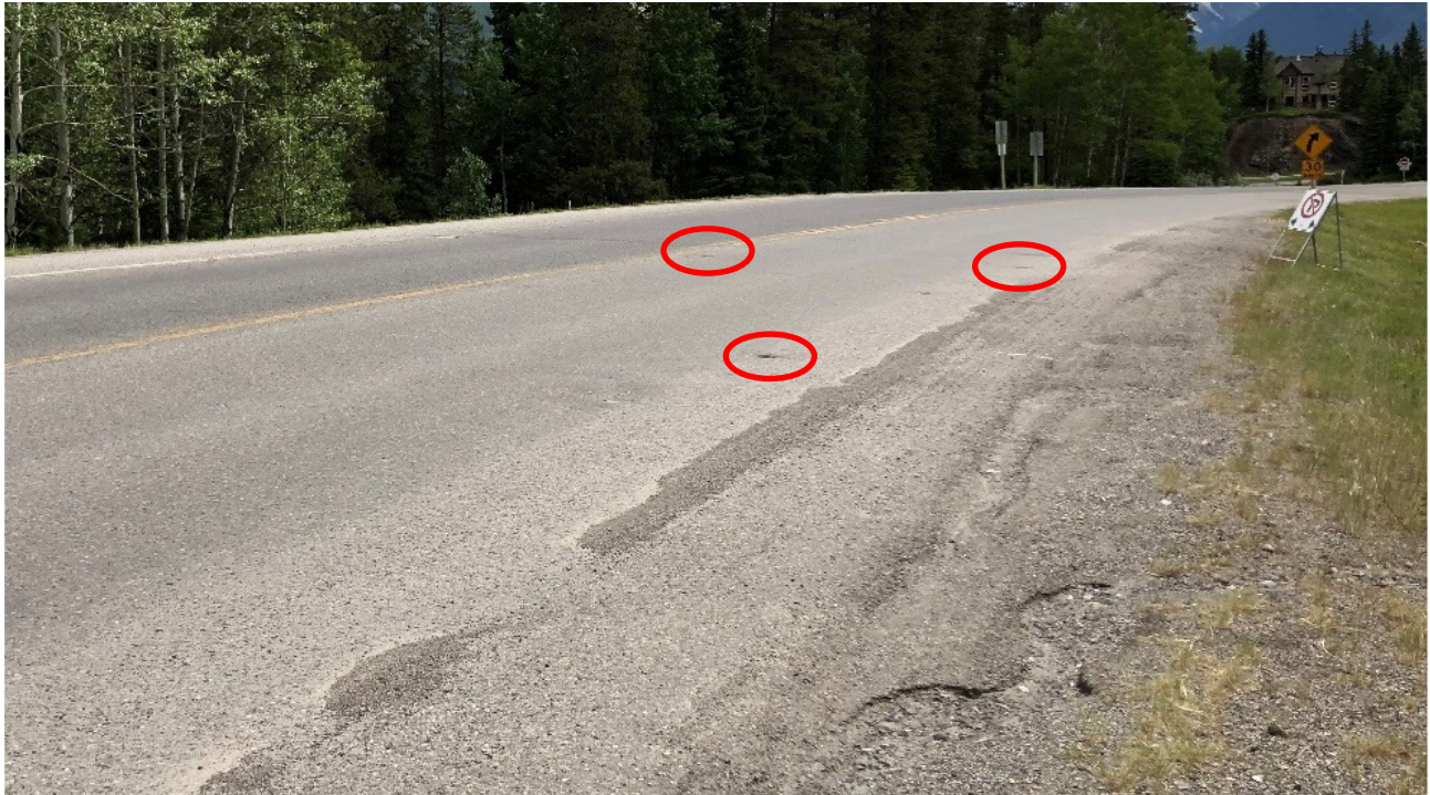
Photo 2 Pavement cracking and flush-mounted headbox for old boreholes. Photo taken facing west on July 6, 2020.
