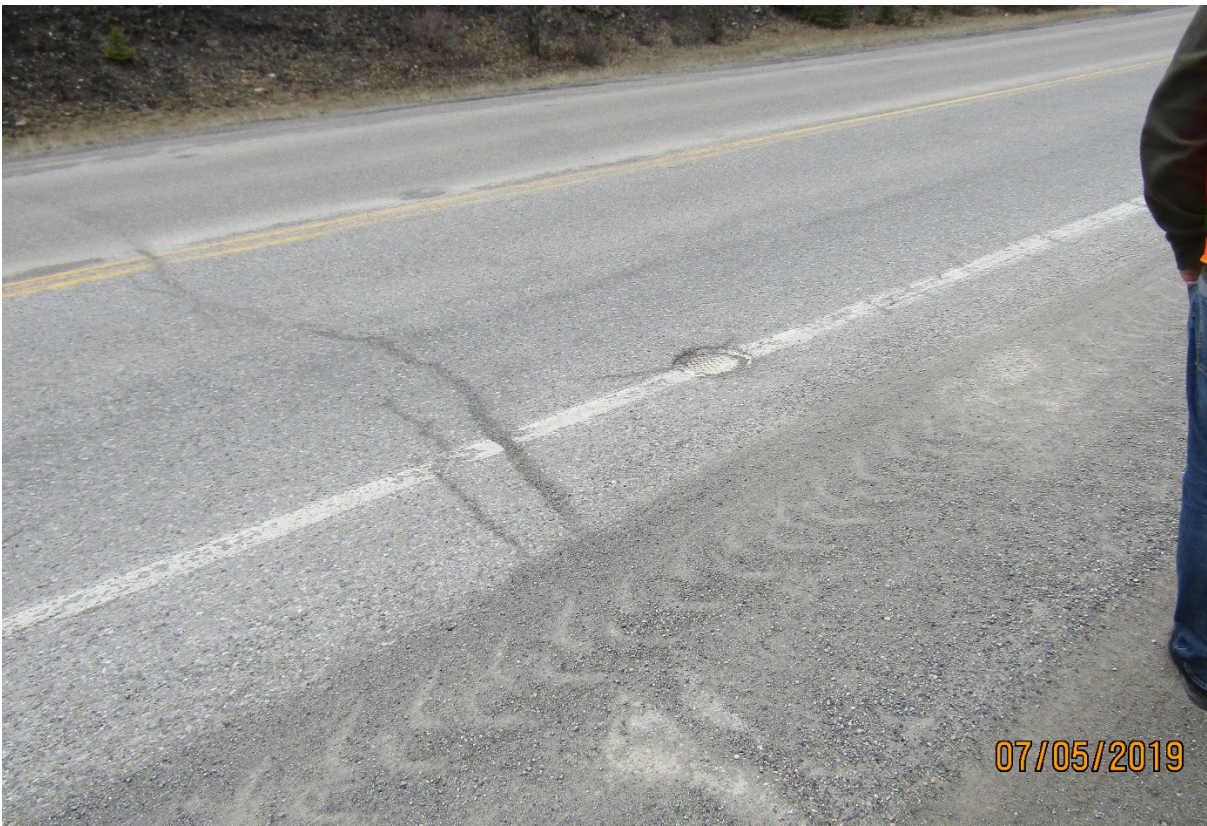
Photo 2 Pavement cracking and flush-mounted headbox for an old borehole. Photo taken facing west on May 7, 2019.
