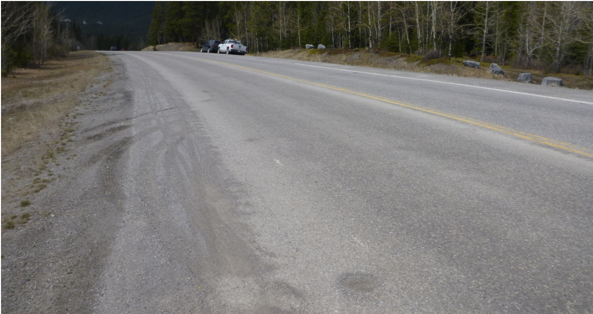
Photo 2 Pavement cracking and flush-mounted headbox for an old borehole. Photo taken facing west on May 7, 2019.
