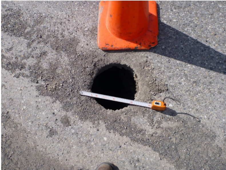
Photo 6 Photo of sinkhole site taken during 2016 Section B inspection. Note that borehole at the location of the sinkhole had a removeable metal cap.
