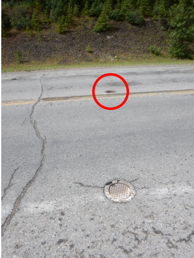
Photo 6 Photo of sinkhole site taken during 2016 Section B inspection. Note that borehole at the location of the sinkhole had a removeable metal cap.
