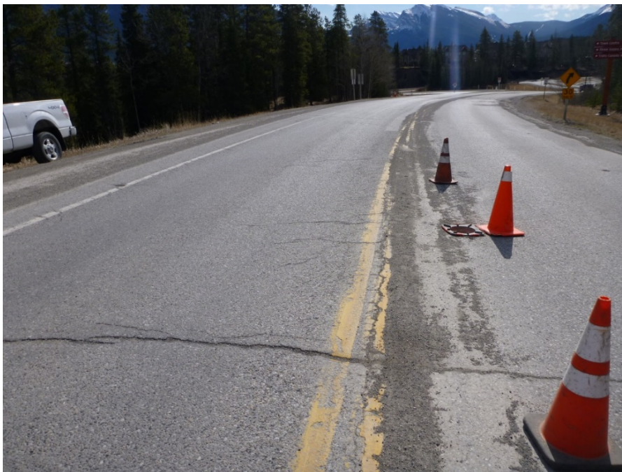
Photo 4 Inverted traffic cone marks location of sinkhole. Photo taken facing southeast.
