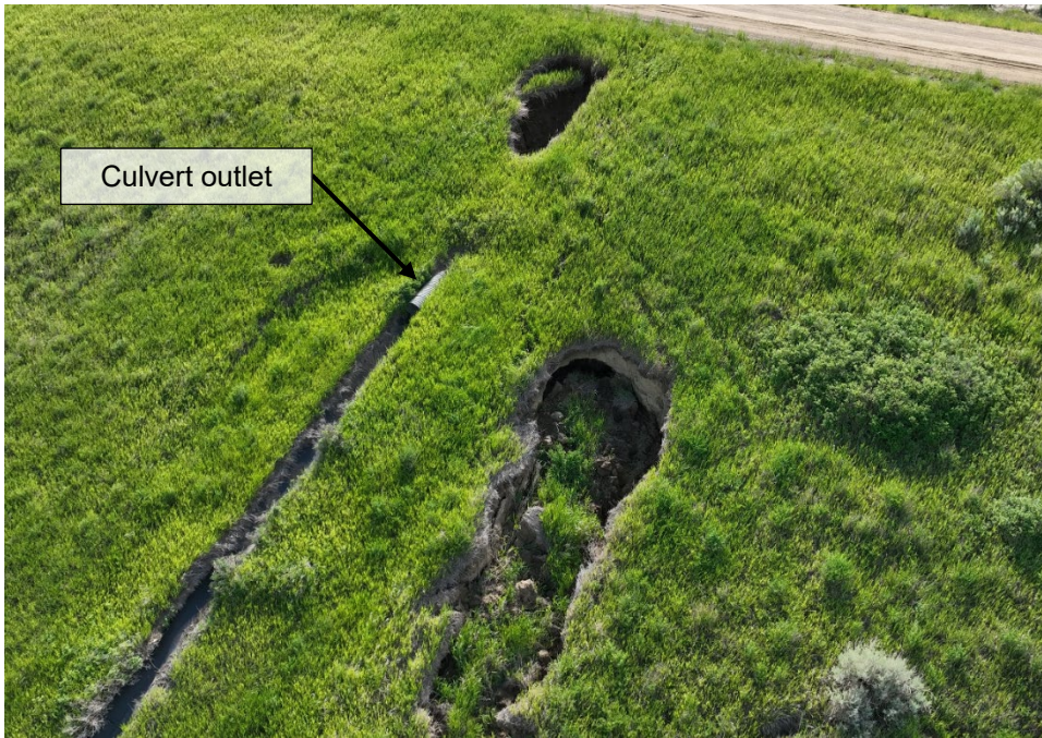
Photo 8 Sinkhole above the culvert and upslope of the slope drain. Sinkhole is approximately 4 m in diameter and up to 2 m to 3 m deep. Lower sinkhole location indicated by black arrow. Photo taken June 18, 2024, facing north.
