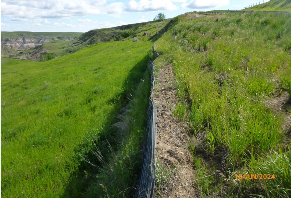
Photo 6 The highway surface is in good condition. There is minor erosion along the south (eastbound) ditch. Photo taken June 18, 2024, facing west.
