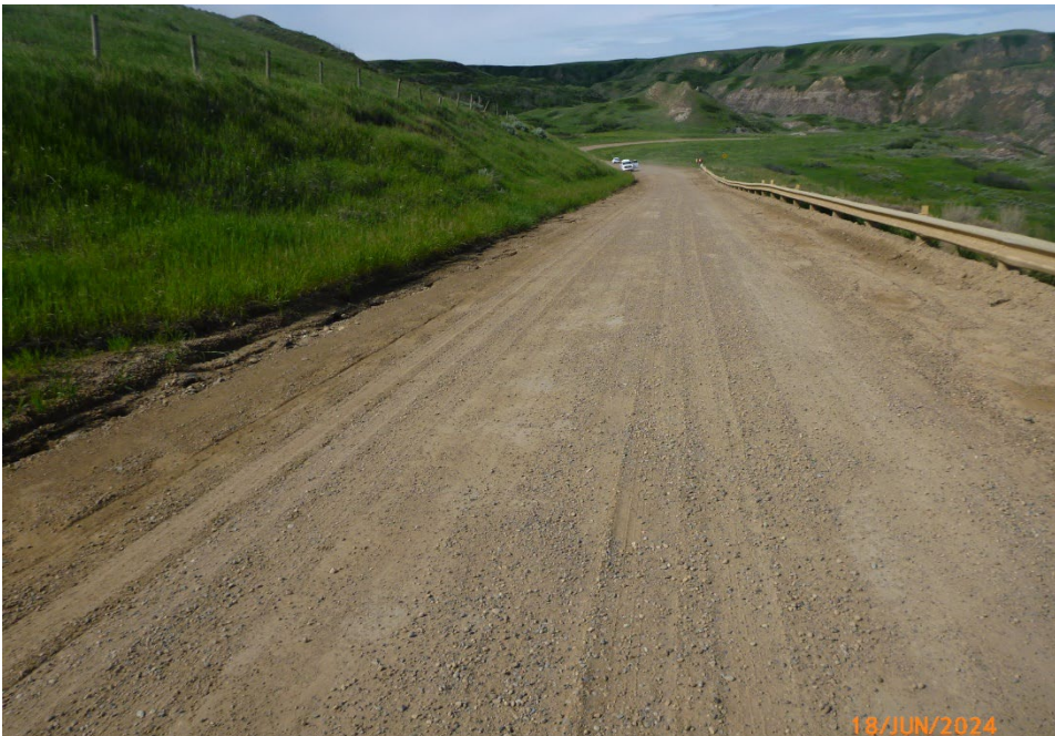
Photo 6 The highway surface is in good condition. There is minor erosion along the south (eastbound) ditch. Photo taken June 18, 2024, facing west.
