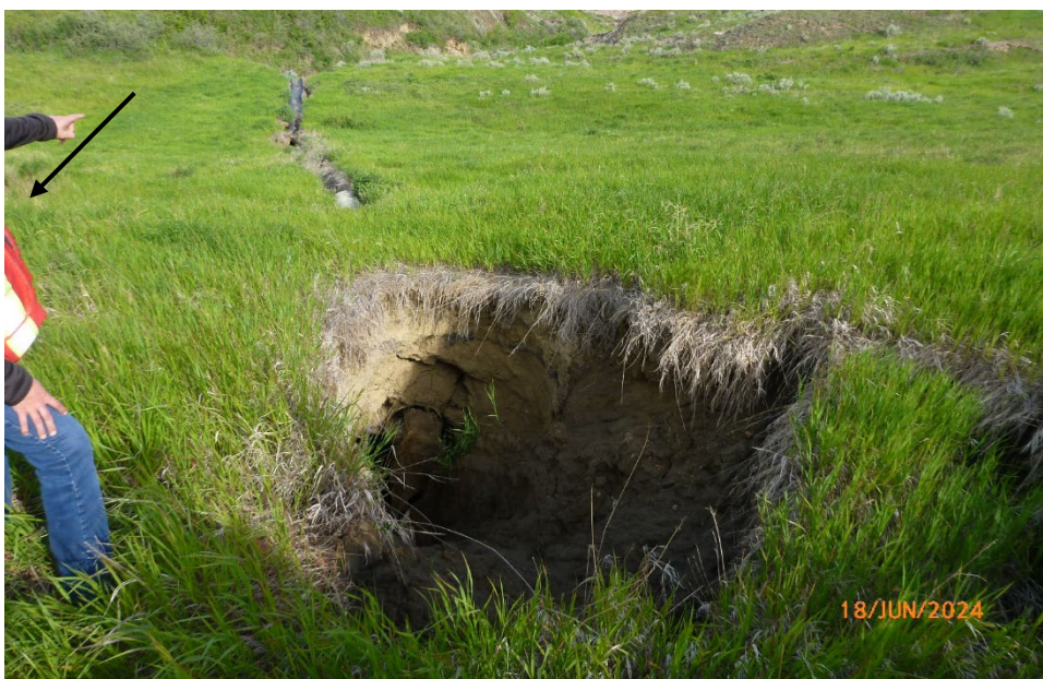
Photo 8 Sinkhole above the culvert and upslope of the slope drain. Sinkhole is approximately 4 m in diameter and up to 2 m to 3 m deep. Lower sinkhole location indicated by black arrow. Photo taken June 18, 2024, facing north.
