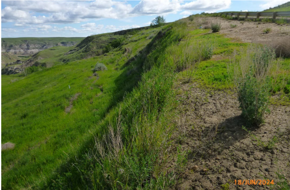
Photo 4 Ground crack up to approximately 50 mm wide located upslope of the geosynthetically reinforced soil wall. Photo taken June 18, 2024.
