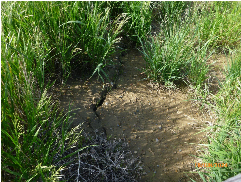
Photo 4 Ground crack up to approximately 50 mm wide located upslope of the geosynthetically reinforced soil wall. Photo taken June 18, 2024.
