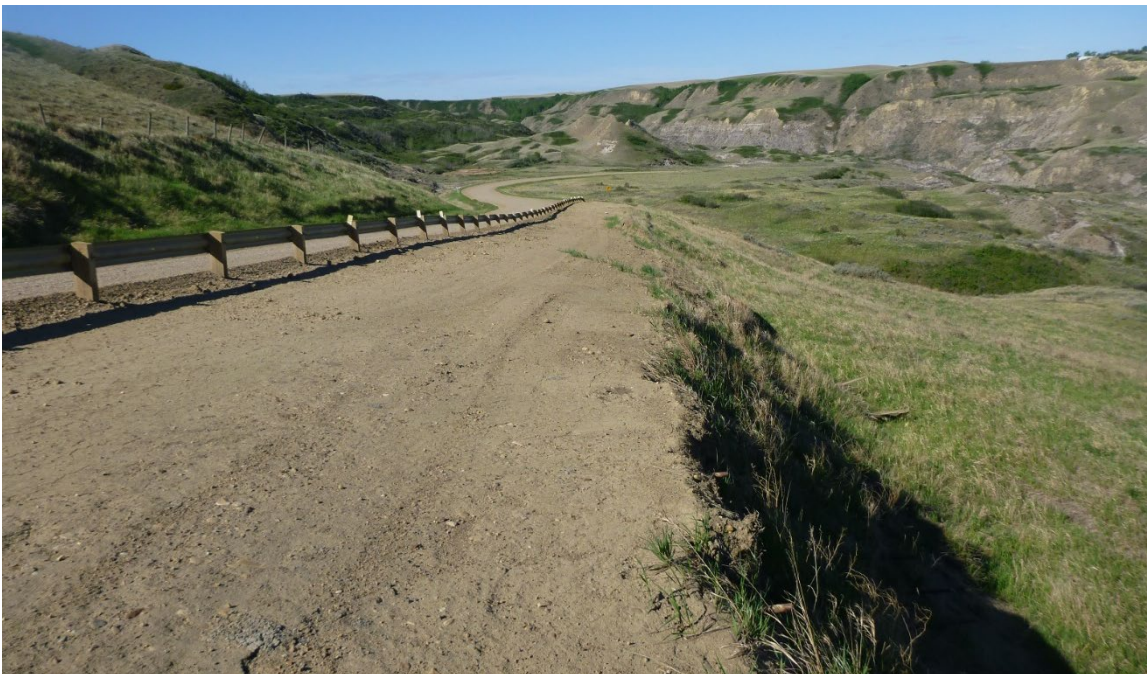
Photo 3 North side of the guardrail has been graded but does not have any vegetation cover. Photo taken May 31, 2022, facing southwest.
