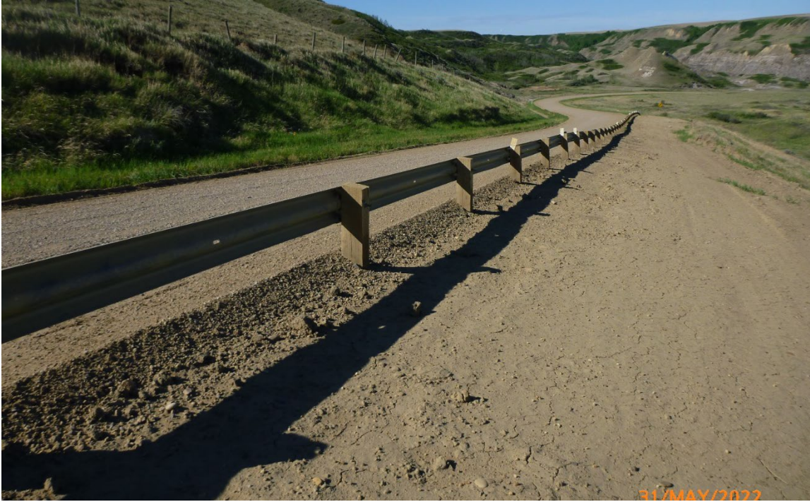
Photo 3 North side of the guardrail has been graded but does not have any vegetation cover. Photo taken May 31, 2022, facing southwest.
