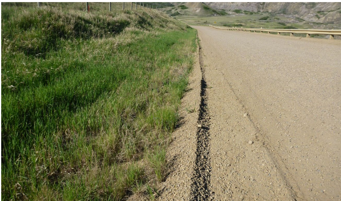
Photo 5 The south (eastbound) ditch was narrowed during the highway realignment and is now a v-ditch. Photo taken May 31, 2022, facing southwest.
