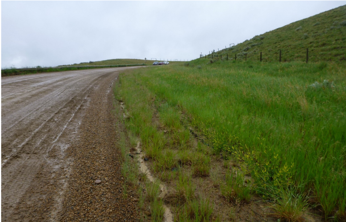
Photo 4 Surface runoff discharges northwards across the road onto the slide mass due to insufficient capacity in ditch on south side of highway. Photo taken facing southwest on June 24, 2021.
