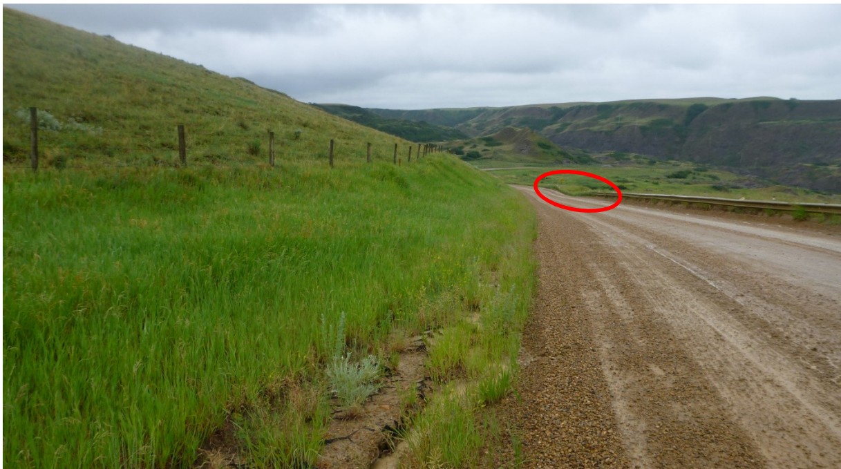
Photo 2 Shallow ditch on south side of highway has insufficient capacity to carry surface flows without discharging water across the road onto the slide mass. Photo taken facing southwest on June 24, 2021.
