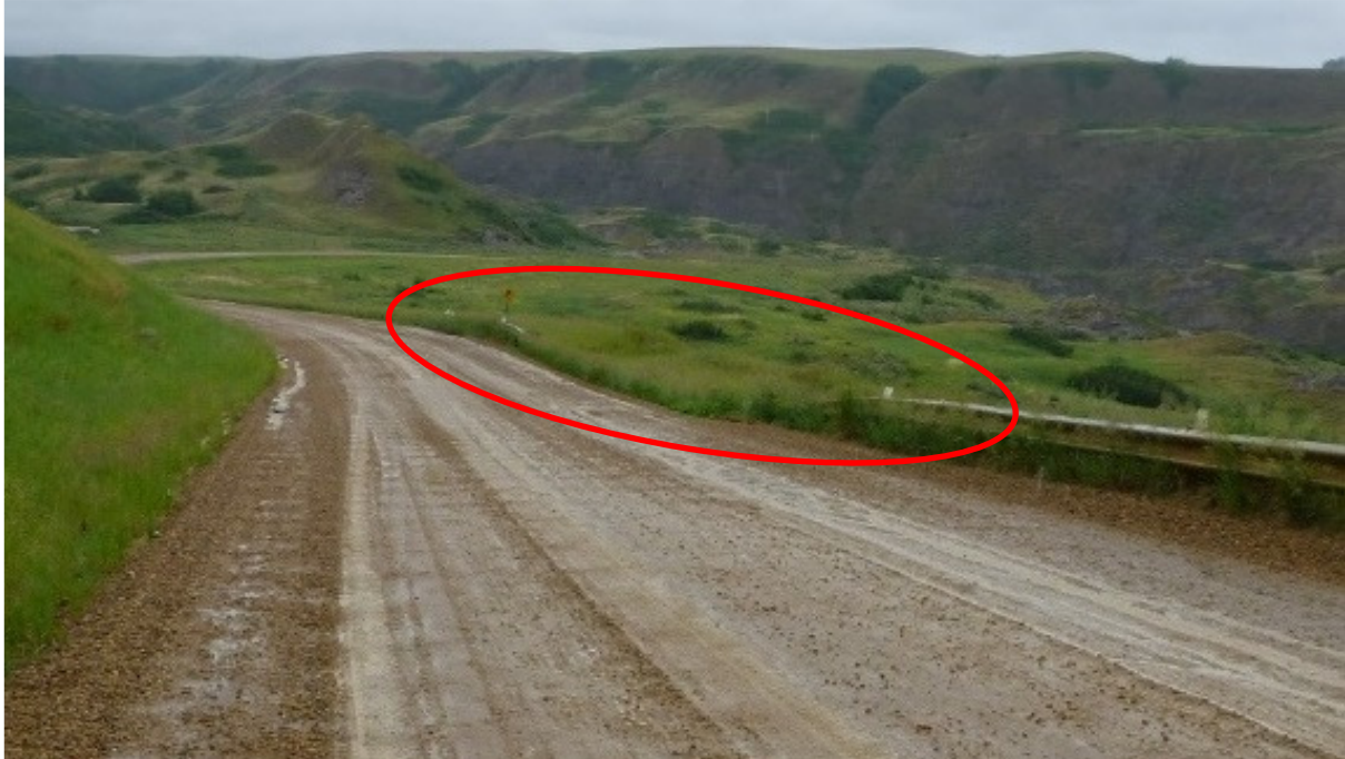
Photo 2 Shallow ditch on south side of highway has insufficient capacity to carry surface flows without discharging water across the road onto the slide mass. Photo taken facing southwest on June 24, 2021.
