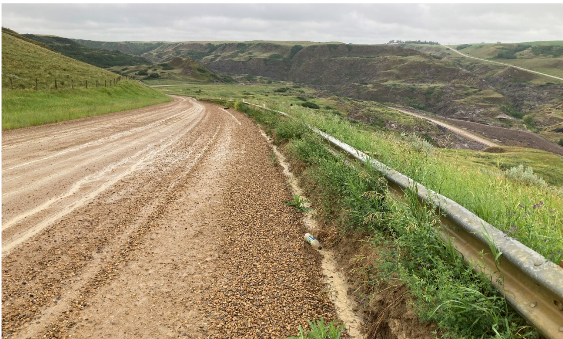
Photo 4 Surface runoff discharges northwards across the road onto the slide mass due to insufficient capacity in ditch on south side of highway. Photo taken facing southwest on June 24, 2021.
