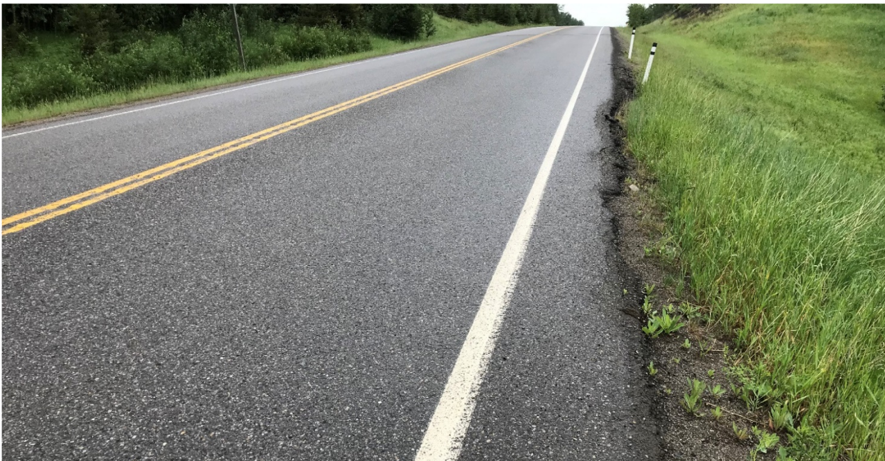
Photo 4 No pavement cracking observed on the highway. Photo taken facing southwest on July 5, 2021.
