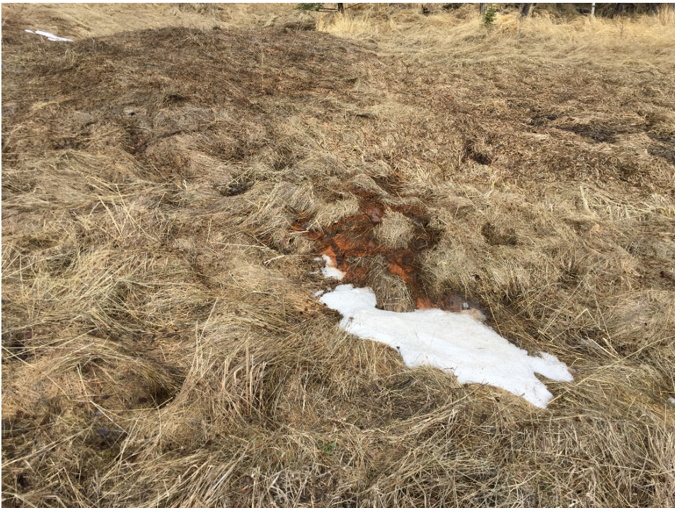
Photo 4 Rust staining from seepage through plugged culvert at the toe of the slide. Photo taken on April 30, 2018.
