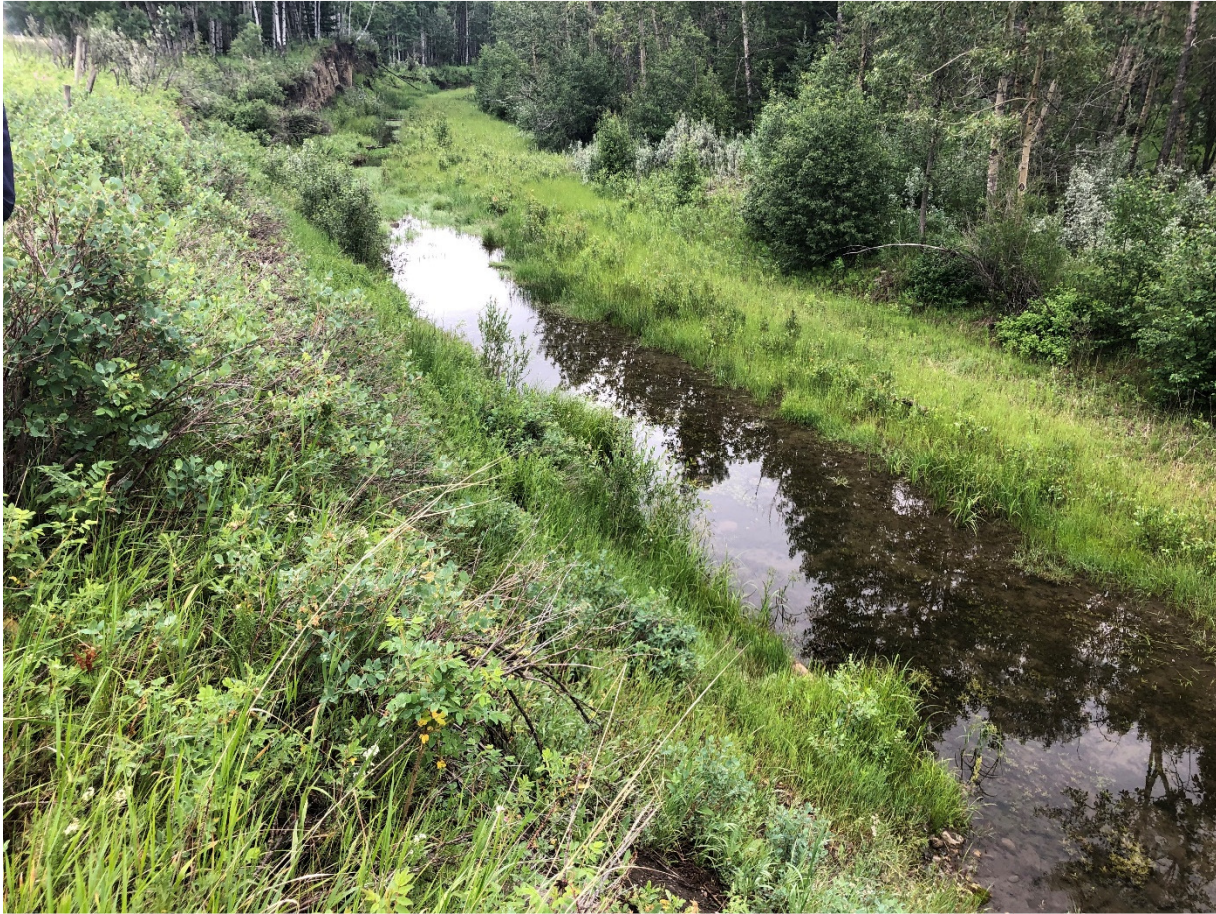
Photo 3 Increased flow in the side channel potentially leading to an increase in bank erosion adjacent to the highway. Photo was taken facing east on July 5, 2021.
