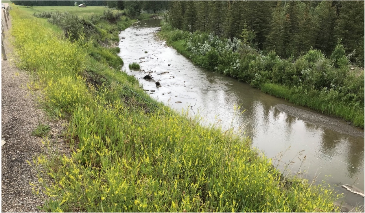
Photo 3 Displaced grass and soil due to surface runoff and ongoing bank erosion from Fisher Creek. Photo taken facing east on July 5, 2021.
