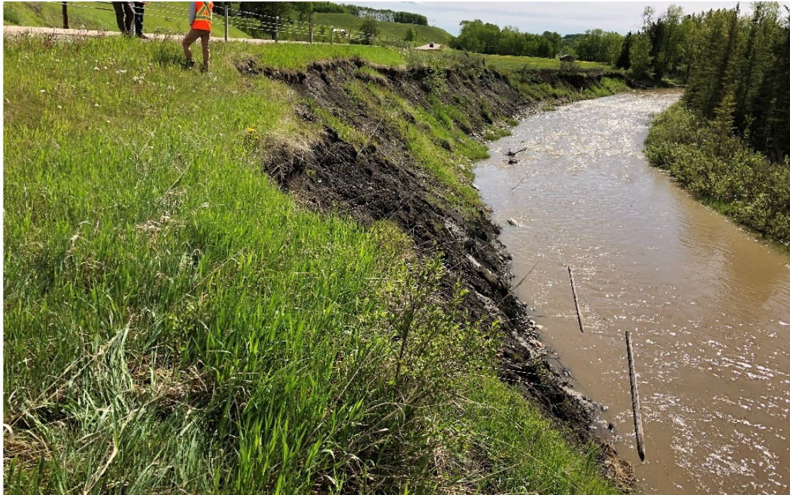
Photo 2 Active slope erosion from creek flow. Photo was taken facing west on June 8, 2020.
