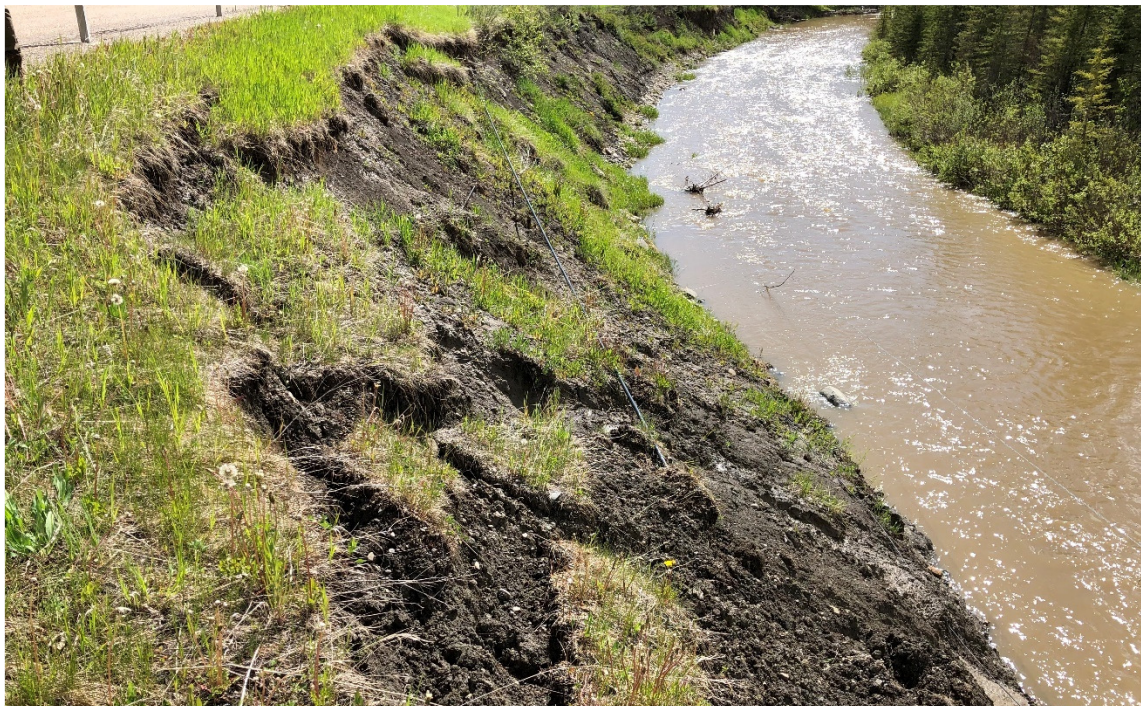
Photo 4 Displaced grass and soil due to surface runoff and ongoing bank erosion from Fisher Creek. Photo taken facing east on June 8, 2020.
