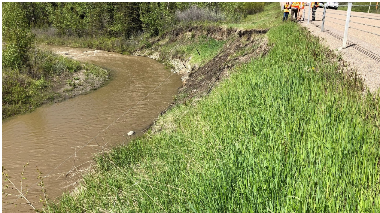
Photo 2 Active slope erosion from creek flow. Photo was taken facing west on June 8, 2020.
