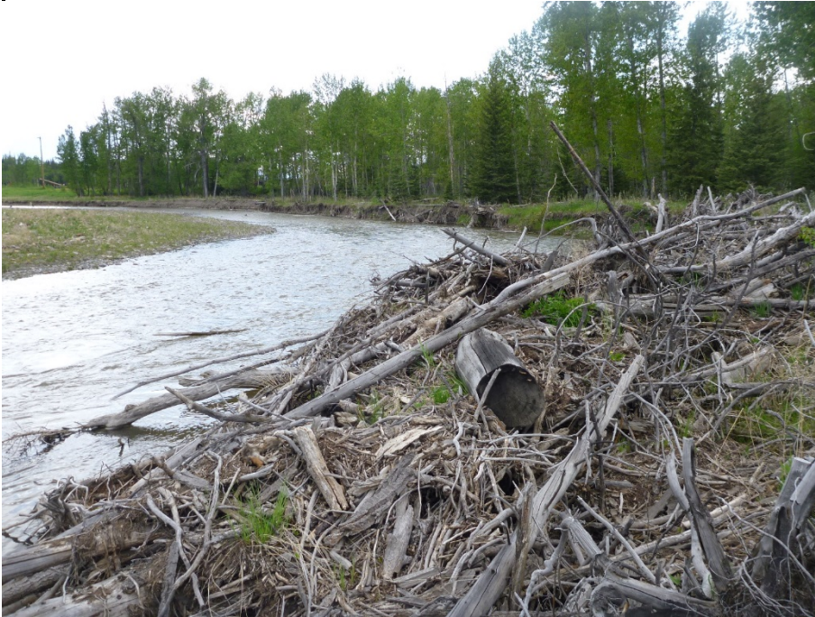
Photo 3 Tree debris blocking river from entering creek. No change in tree debris from 2016 inspection. Some additional plant growth. Photo was taken facing southwest on May 29, 2017.
