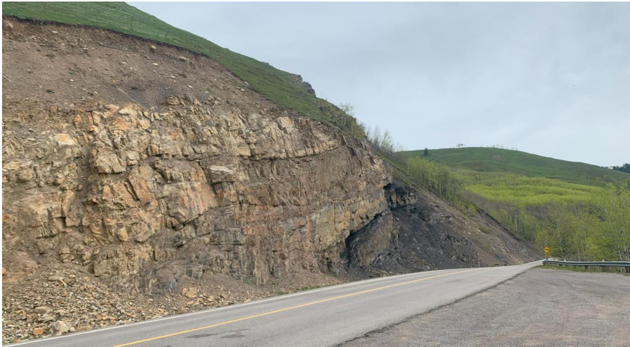
Photo 2 Rock slope north of highway. Coal seams creating rock overhang on slope. Photo was taken facing northwest on May 28, 2024.
