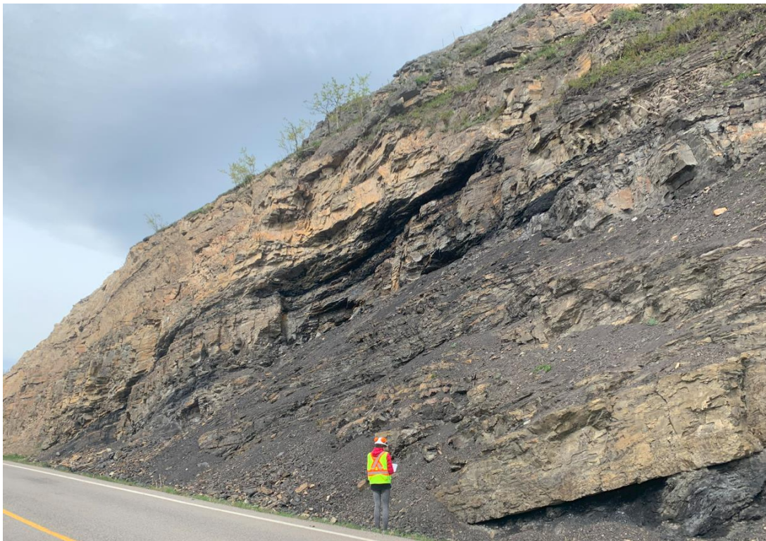
Photo 2 Rock slope north of highway. Coal seams creating rock overhang on slope. Photo was taken facing northwest on May 28, 2024.
