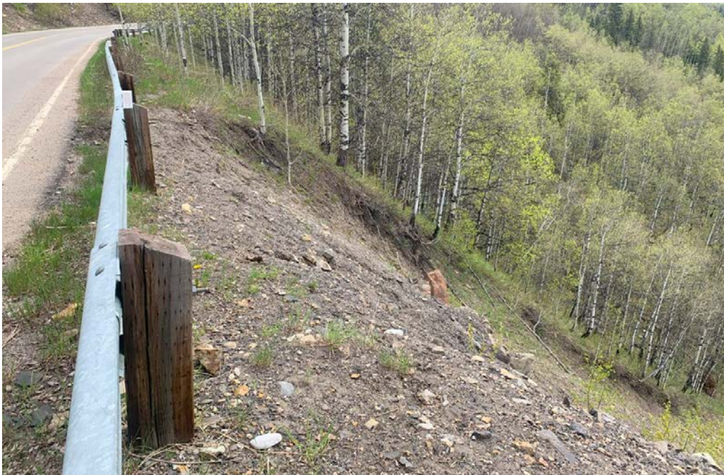
Photo 6 Surface runoff erosion on the south side of highway has undermined the guardrail and reached the pavement edge. There was no evidence of pavement crack during the 2024 inspection. Photo taken facing east on May 28, 2024.
