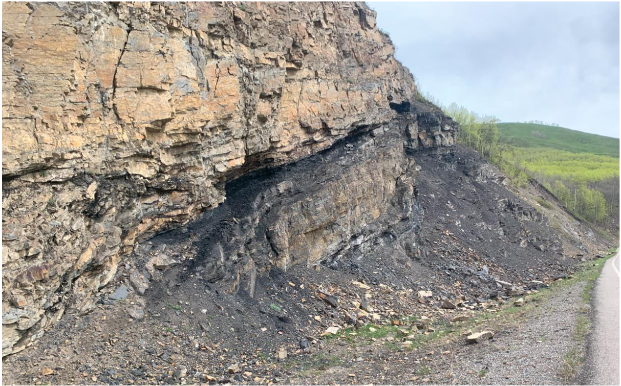
Photo 4 Rock blocks in the ditch on the north side of the highway. Photo taken on May 28, 2024.
