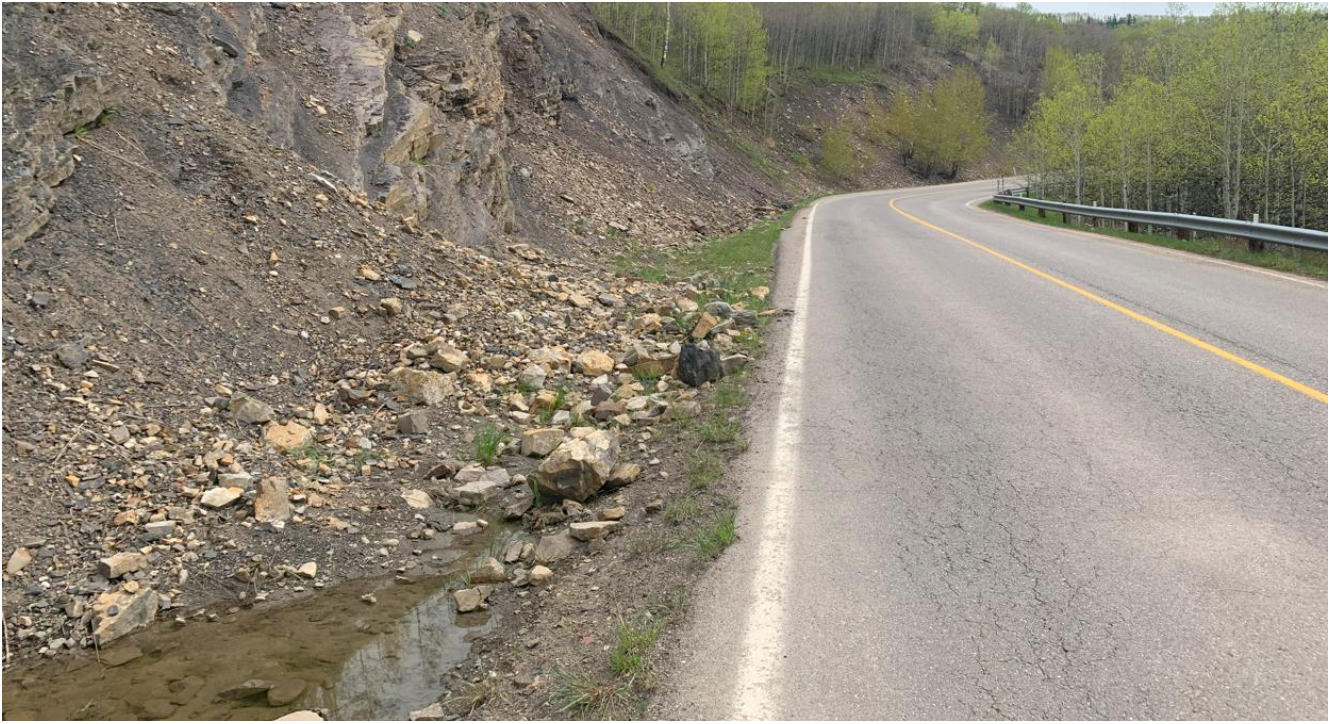
Photo 6 Surface runoff erosion on the south side of highway has undermined the guardrail and reached the pavement edge. There was no evidence of pavement crack during the 2024 inspection. Photo taken facing east on May 28, 2024.
