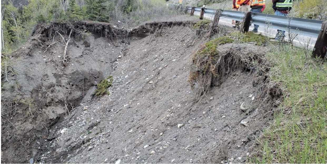
Photo 4 Failure of slope close to the shoulder of the eastbound lane, undermining guardrail post. Photo taken May 28, 2024, facing southwest.
