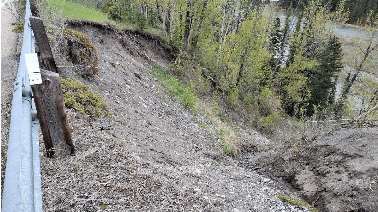
Photo 2 View from highway of the erosion gully, facing downslope. An alluvial fan is forming in the Sheep River due to ongoing erosion. Photo taken May 28, 2024, facing south.
