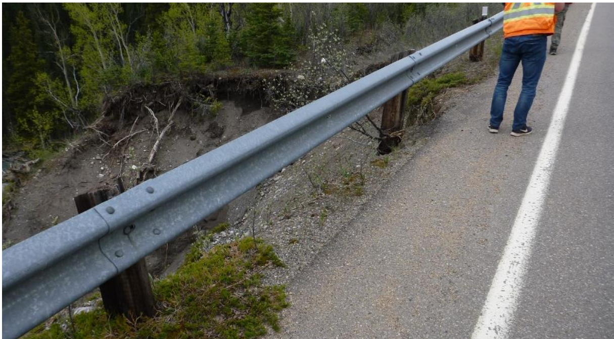
Photo 4 Failure of slope close to the shoulder of the eastbound lane, undermining guardrail post. Photo taken May 28, 2024, facing southwest.
