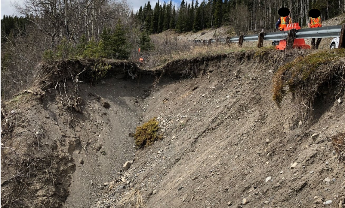
Photo 4 Slumping of the bank on the left (east) flank due to ongoing erosion (indicated by red circle). Photo taken May 16, 2022, facing southwest.
