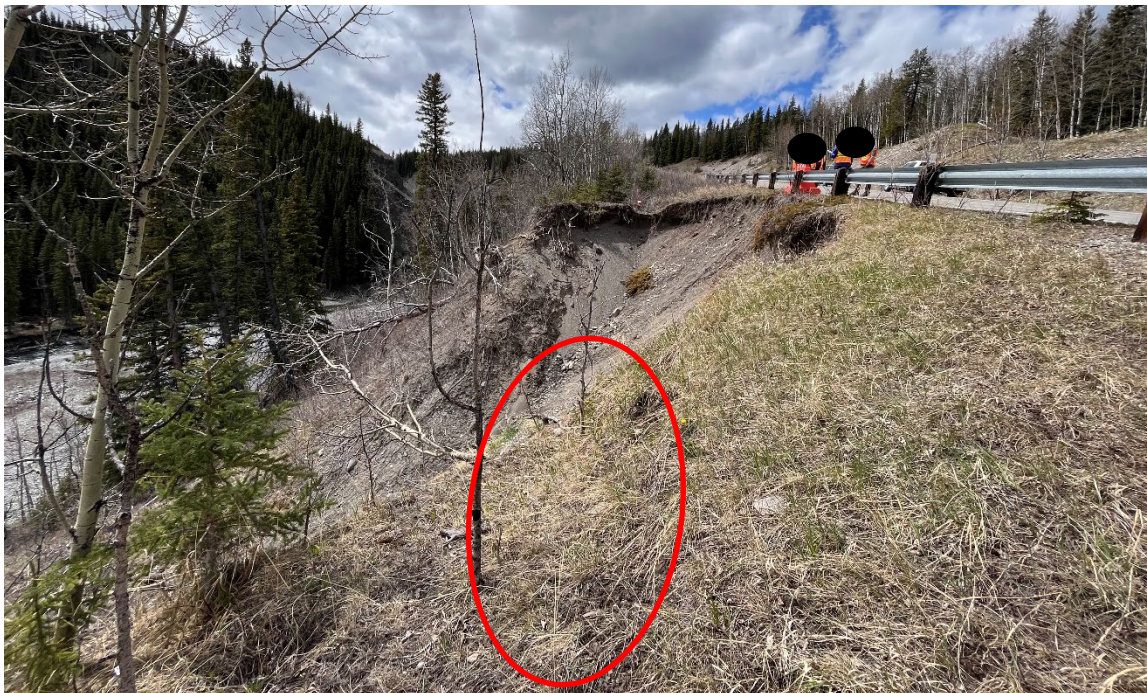
Photo 4 Slumping of the bank on the left (east) flank due to ongoing erosion (indicated by red circle). Photo taken May 16, 2022, facing southwest.
