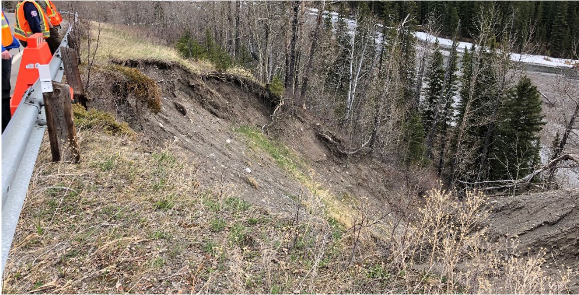
Photo 2 View from highway of the erosion gully, facing downslope. An alluvial fan is forming in the Sheep River due to ongoing erosion. Photo taken May 16, 2022, facing southeast.
