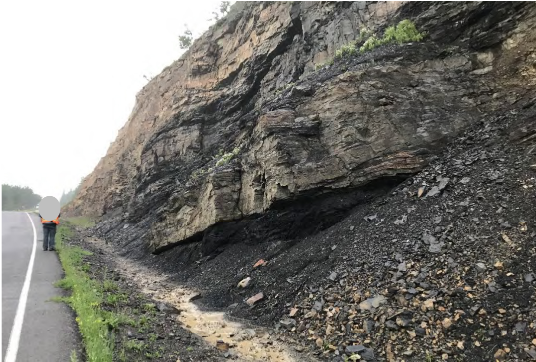
Photo 2 Rock slope north of highway. Rock fall ditch appeared to have been cleaned out recently. Photo was taken facing east on July 5, 2021.
