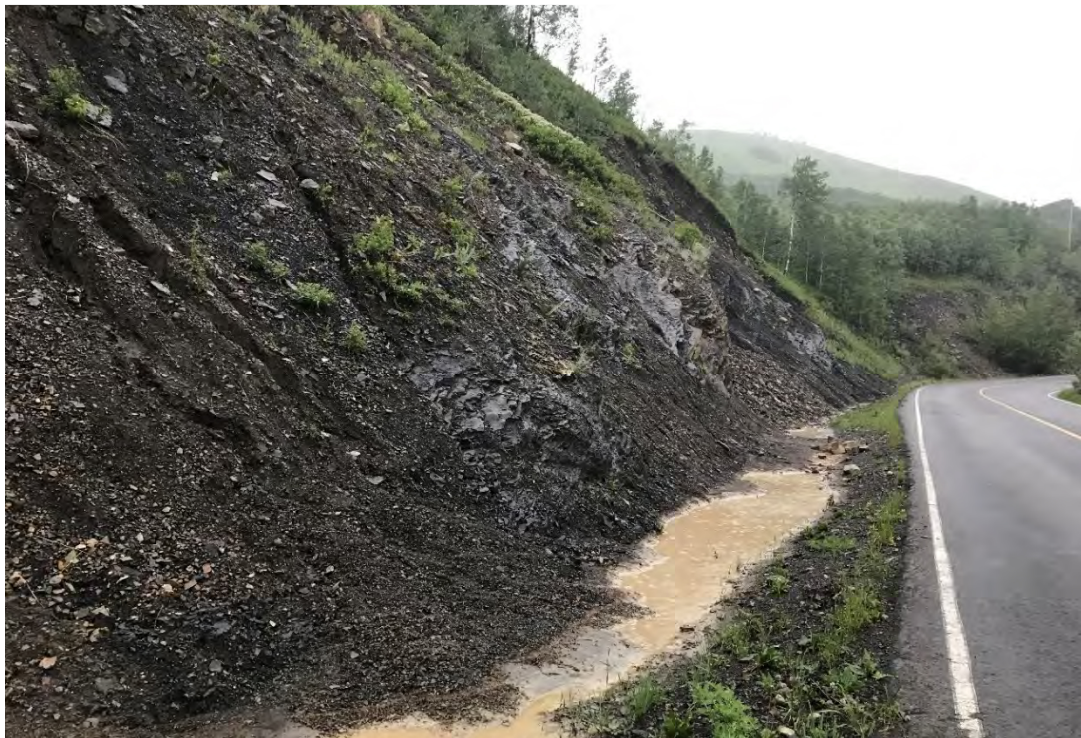
Photo 2 Rock slope north of highway. Rock fall ditch appeared to have been cleaned out recently. Photo was taken facing east on July 5, 2021.
