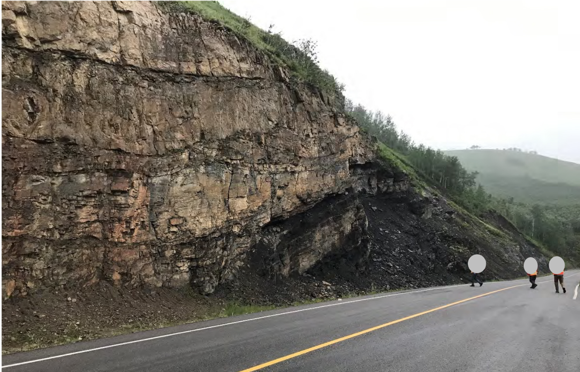
Photo 4 Rock block in the ditch on the north side of the highway. Photo taken on July 5, 2021.
