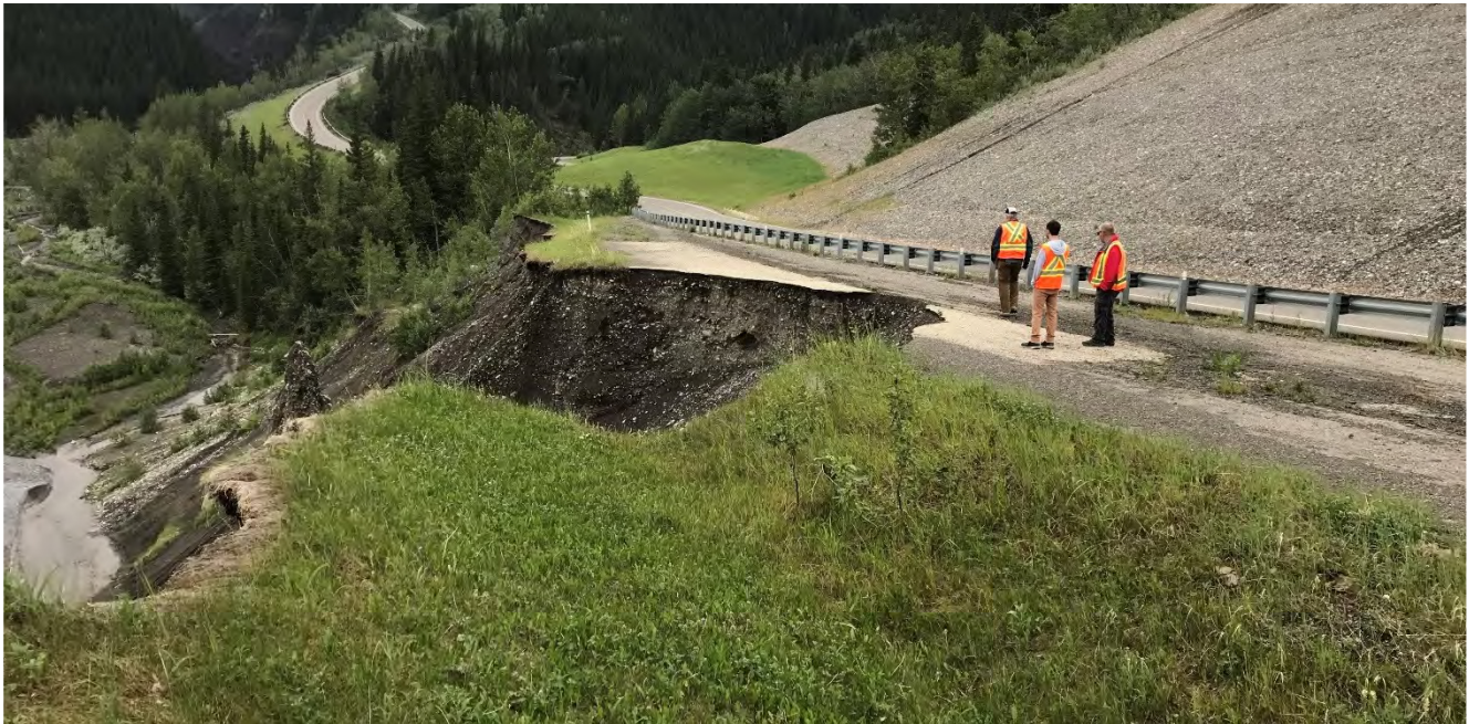
Photo 2 Ongoing slope retrogression. Photo was taken facing south on July 5, 2021.
