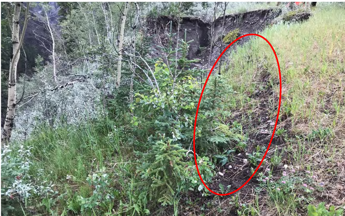
Photo 4 Slumping of the bank on the left flank due to ongoing erosion. Photo taken facing northwest on July 5, 2021.
