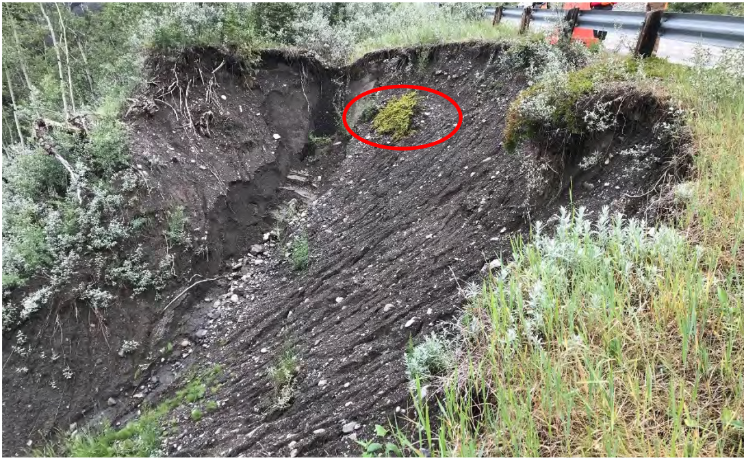
Photo 4 Slumping of the bank on the left flank due to ongoing erosion. Photo taken facing northwest on July 5, 2021.
