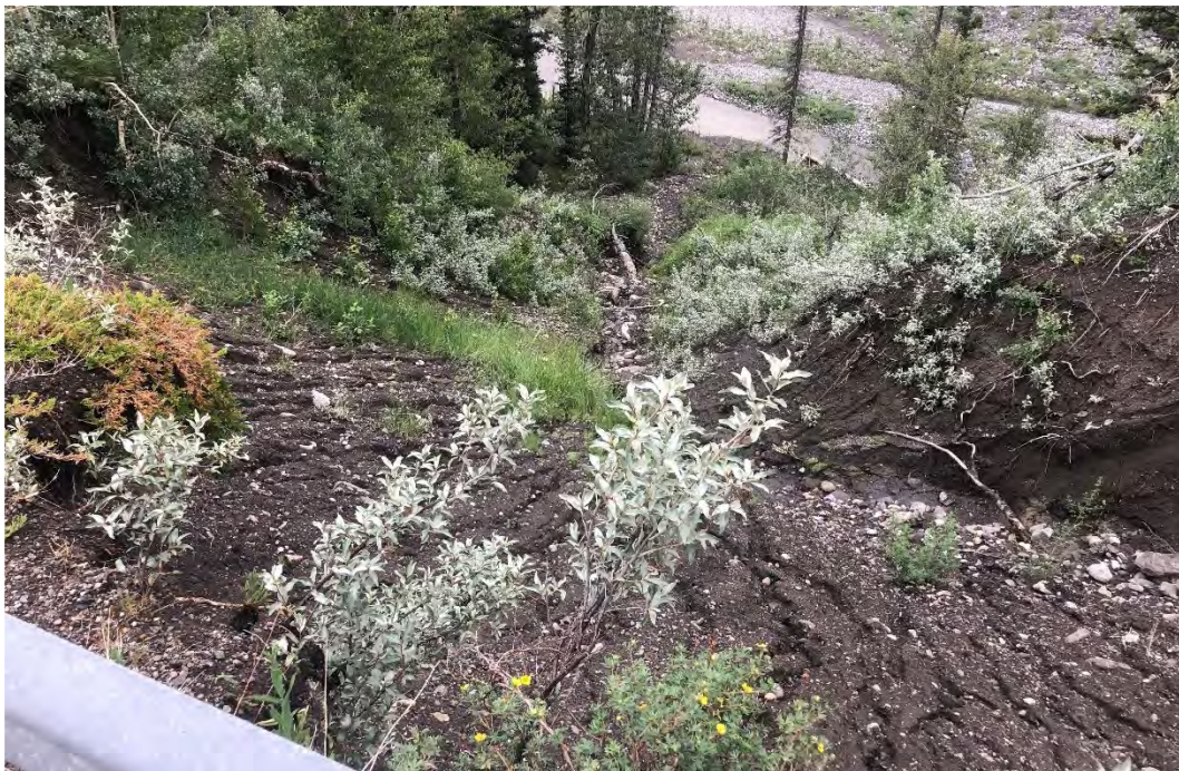
Photo 2 View from highway down the erosion gully. An alluvial fan is forming in the Sheep River due to erosion. Photo taken facing southeast on July 5, 2021.
