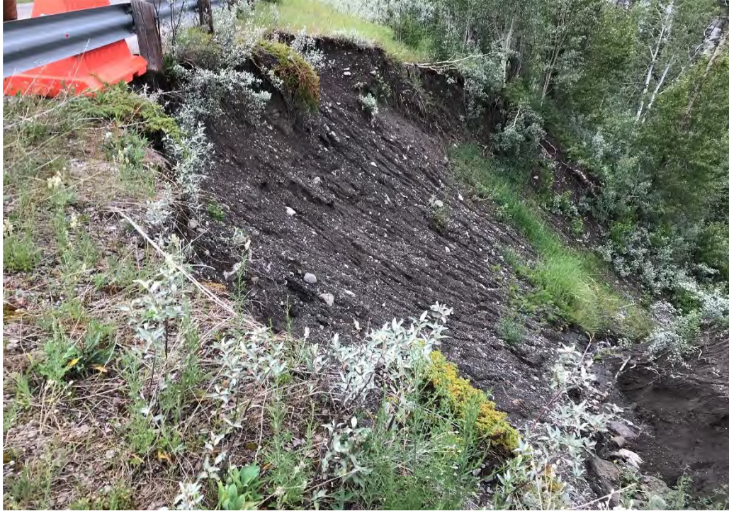
Photo 2 View from highway down the erosion gully. An alluvial fan is forming in the Sheep River due to erosion. Photo taken facing southeast on July 5, 2021.
