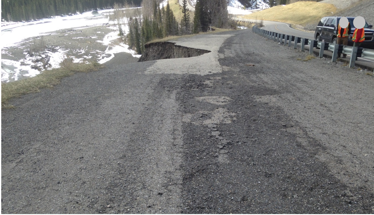
Photo 2 Ongoing slope retrogression. Photo was taken facing west on May 6, 2019.
