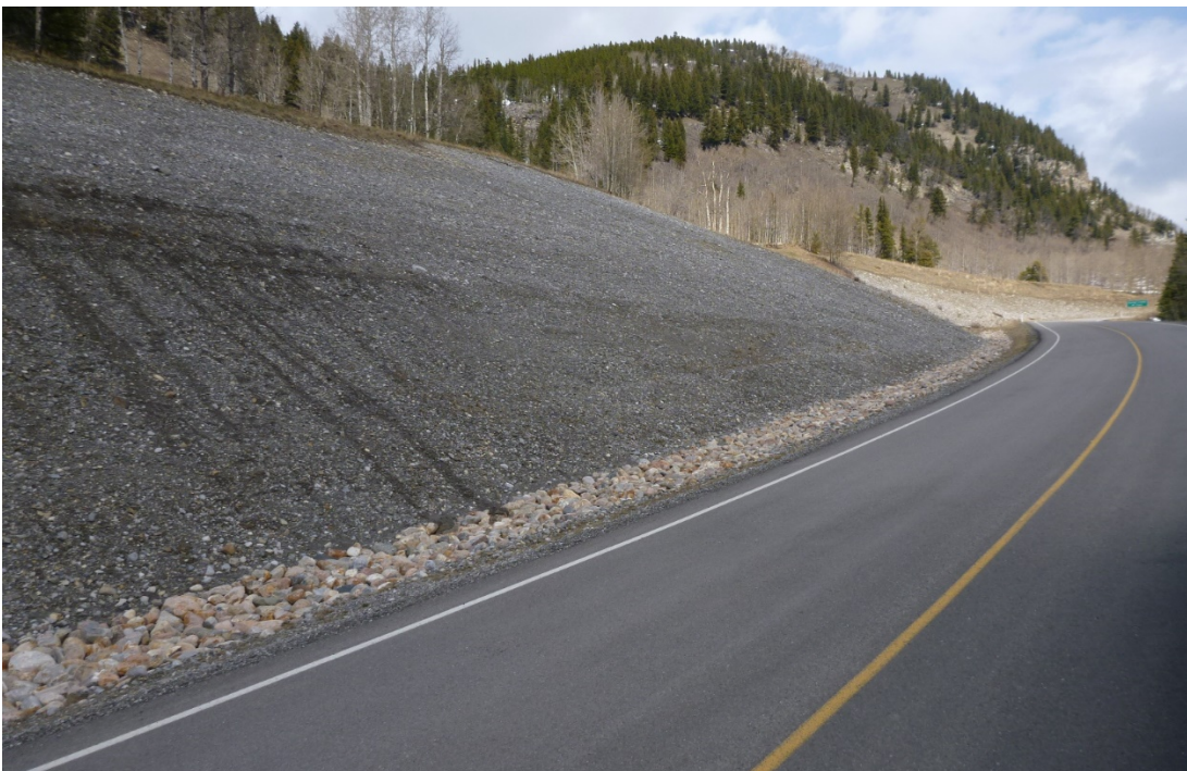
Photo 4 Unvegetated cut slope from highway realignment. Photo was taken facing east on May 6, 2019.
