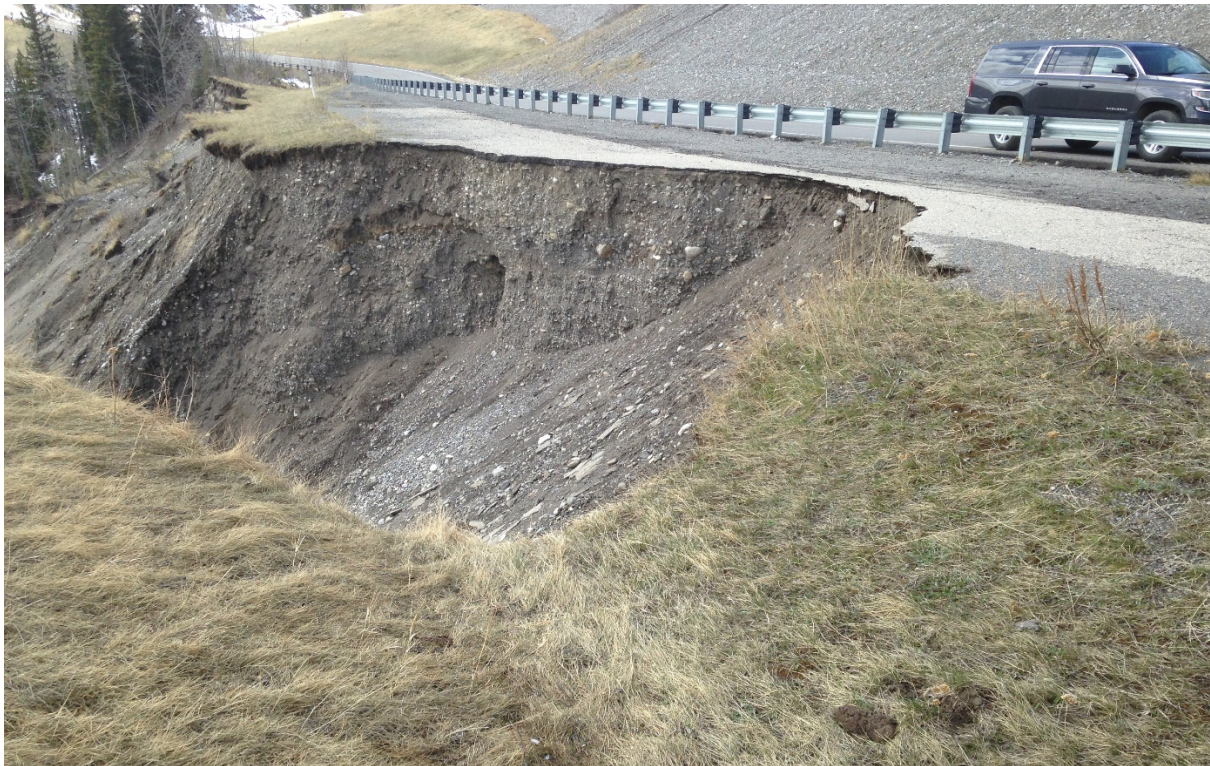
Photo 2 Ongoing slope retrogression. Photo was taken facing west on May 6, 2019.
