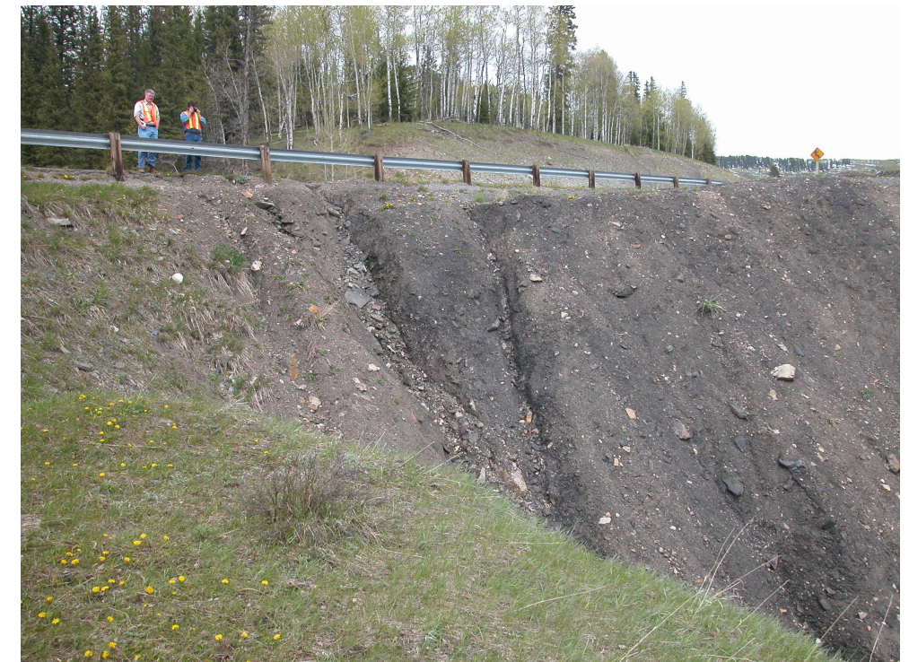
Photo S13-3 (lower left) – May 2004 – facing east across the site, showing the relative position of the gully erosion in the fill embankment slope face and the guardrail/road surface. Note the pile of rockfall debris that has been hauled from a site to the east and stockpiled here for later disposal into the gully downstream of the road.
